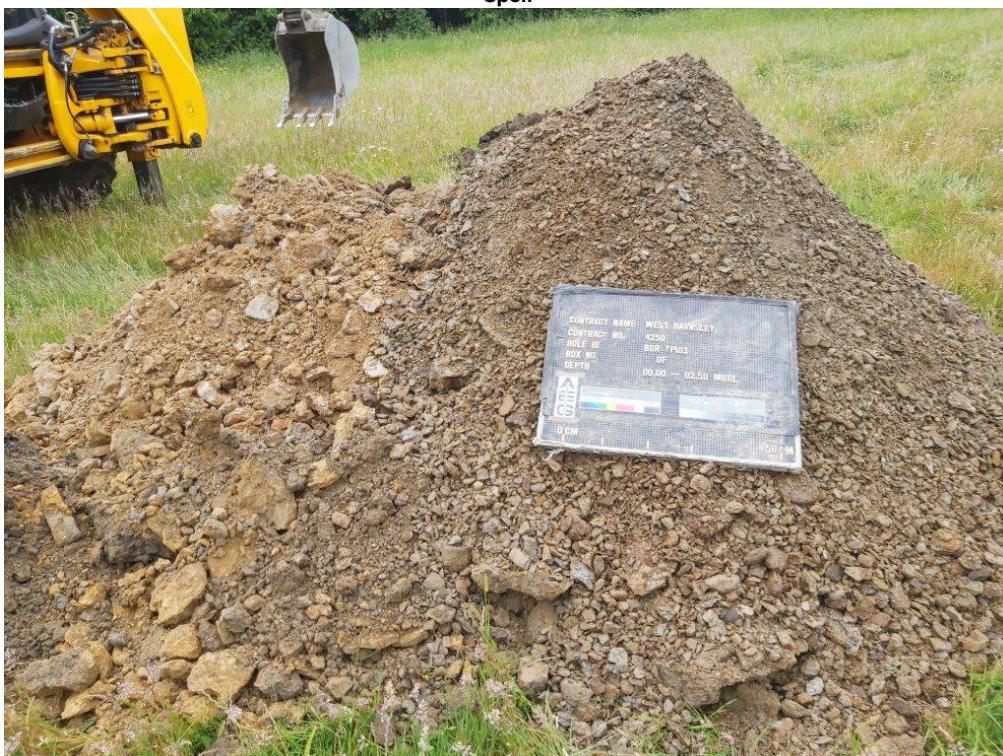
Figure BGR_TP103.4 Spoil
