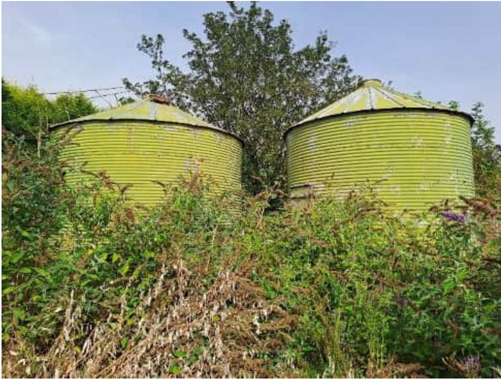
Plate A-3 – Two corrugated metal silos present at the southwestern aspect of the Site. A collection of two corrugated metal silos. One silo removed/ no longer present.
