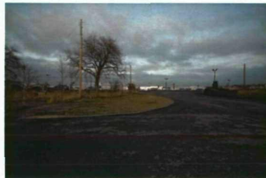
View of the Claycliffe Road access from the site.
