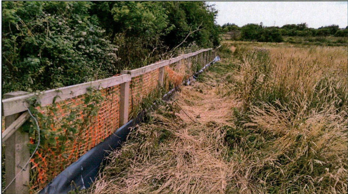
Plate 1: Photograph showing one-way herptile fencing located along the southern, eastern and western boundaries of the Site.
