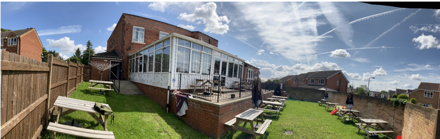
Existing Rear (SW) Elevation to Outside Seating Area (Location for (2no) Proposed Fixed Timber Frame Pergolas, and High Timber Close Boarded Fence)
