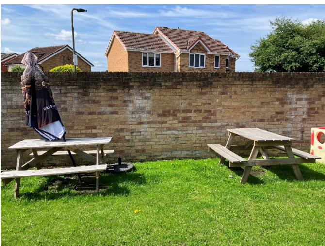
Existing Rear Boundary Wall (SW) Elevation to Chantry Grove (To Remain as Existing)
