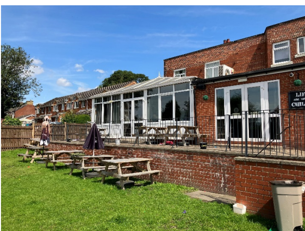
Existing Rear (SW) Elevation to Outside Seating Area (Location for Proposed Fixed Timber Frame Pergola, and High Timber Close Boarded Fence/ New Lightweight Insulated Pitched Roof to Existing Conservatory)
