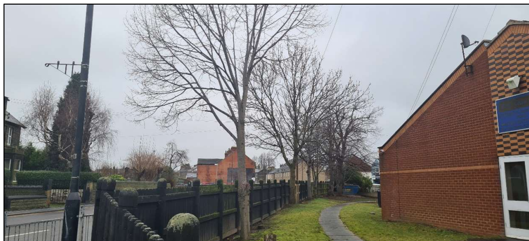
External inspection – care home
