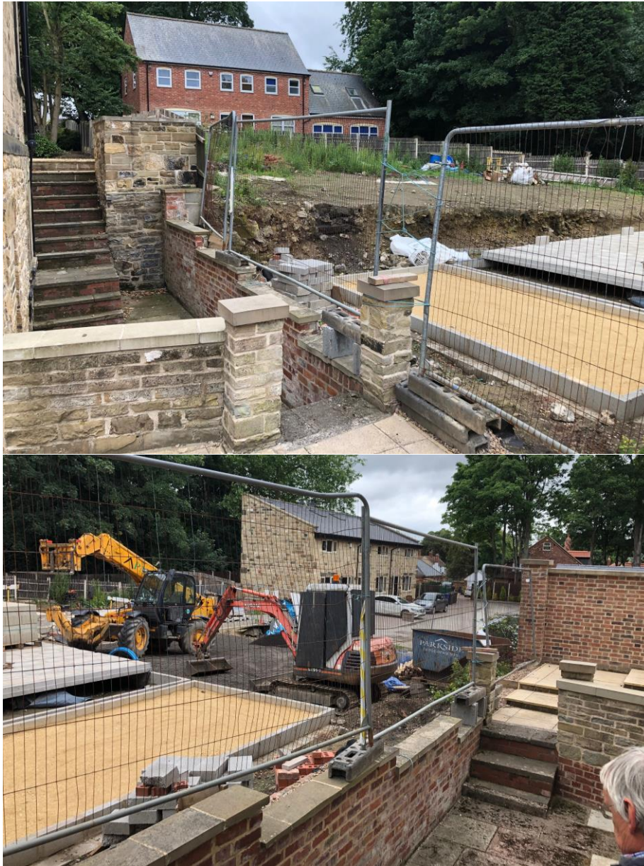
Fig. 8 & Fig. 9 – West Boundary: Random rubble stone wall and stone piers; clay brickwork; pc copings.
