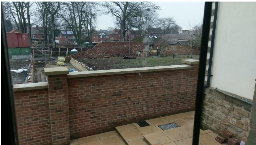
Fig 18 Brick wall adjacent house – new bricks, piers and cappings to match the recently constructed, new short section of wall
