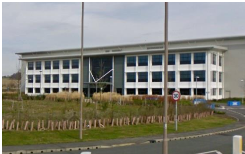
Fig. 5 ASOS office opposite site
