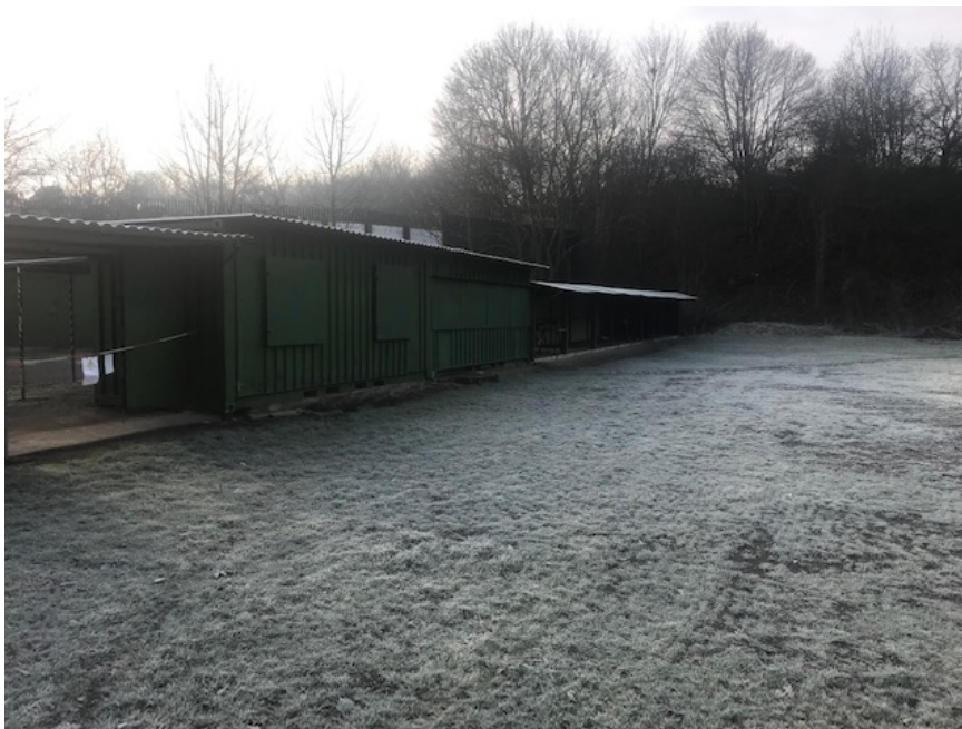
Existing Cabins- used as the shooting points for 50 and 100 yard ranges.
