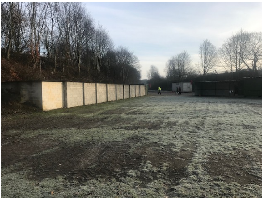
Existing, looking back towards main entrance.
