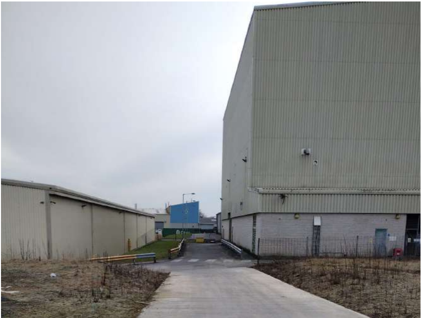
5. View looking east with 30 meter+ tall unit on the right
