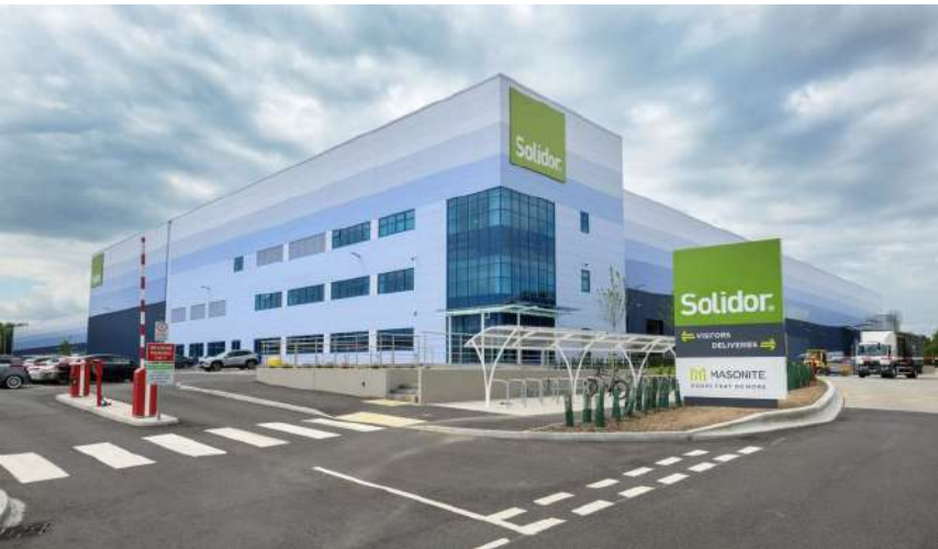
Above is the existing Solidor facility at Stoke-on-Trent which is the sister facility to our Premdor scheme, it was important to the client that both facilities should have a certain level of aesthetic consistency to project a modern outward looking company.
