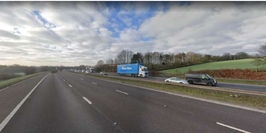
1. View looking south from M1
