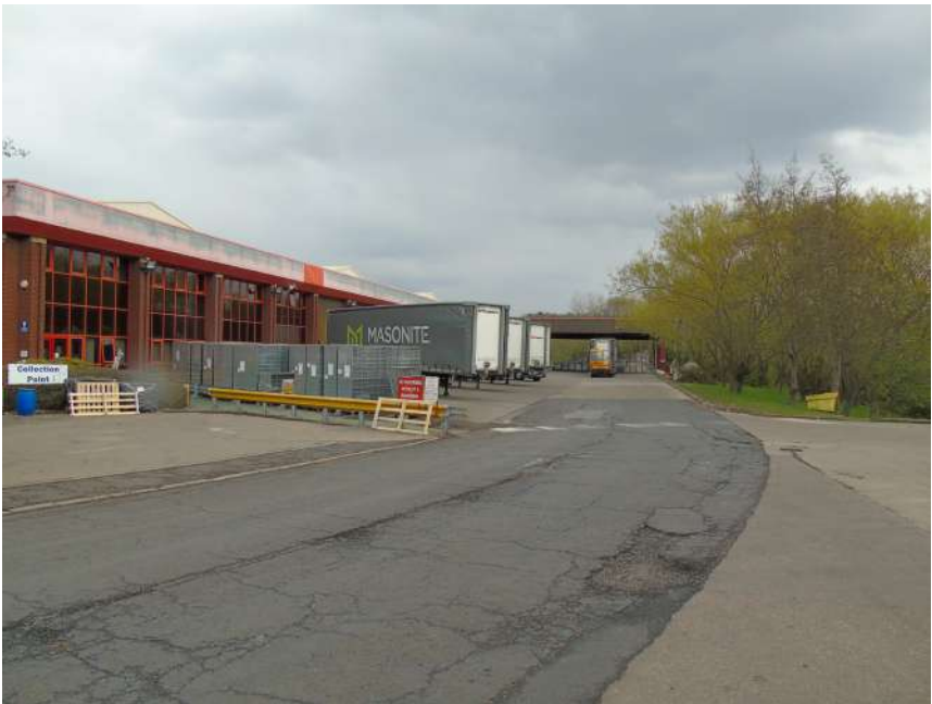
2. View from main access road to western unit
