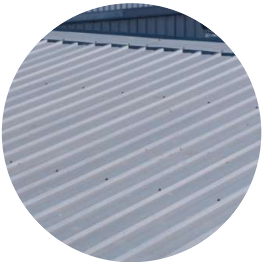
Metal profiled roof
