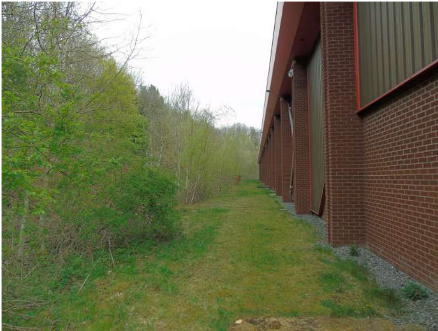
4. View looking north with embankment on left
