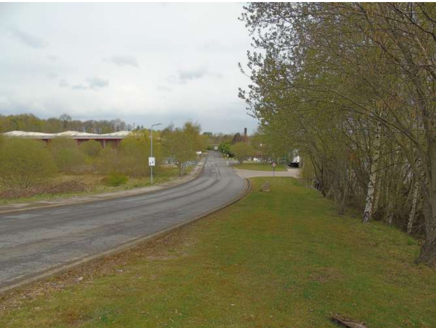
1. View looking north down access road
