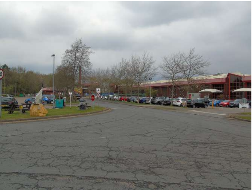
3. View from main access road to Eastern unit
