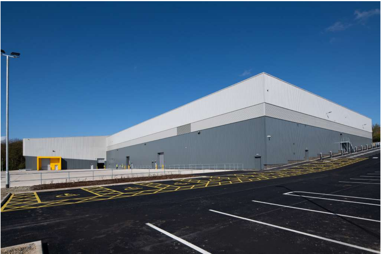
Bradley Business Park Phase III (Afex Hose)
