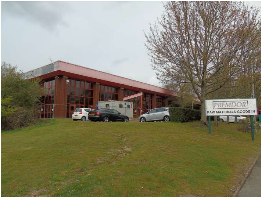
1. View looking north west onto entrance of western unit
