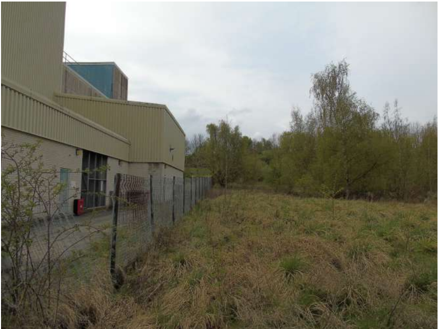
5 . View looking south at site edge
