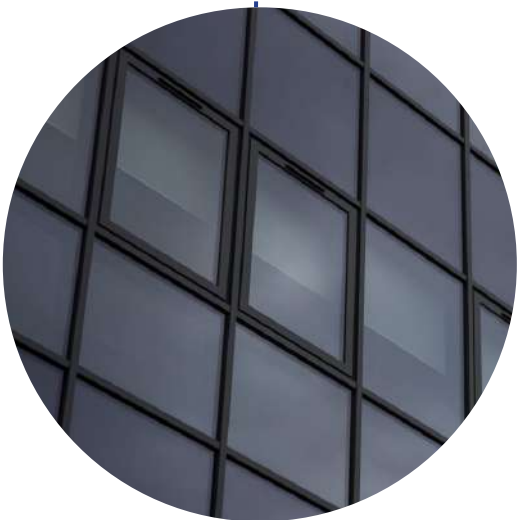
Profiled curtain wall
