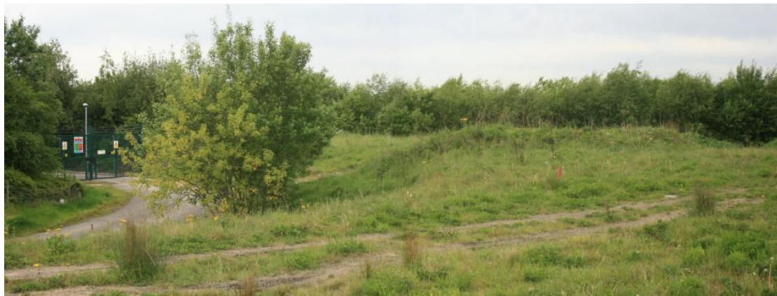
THE SUB-STATION ACCESS OFF THE ROUNDABOUT AT THE SOUTH END OF THE SITE
