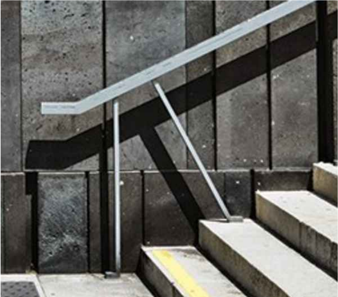
Example Handrail Image
