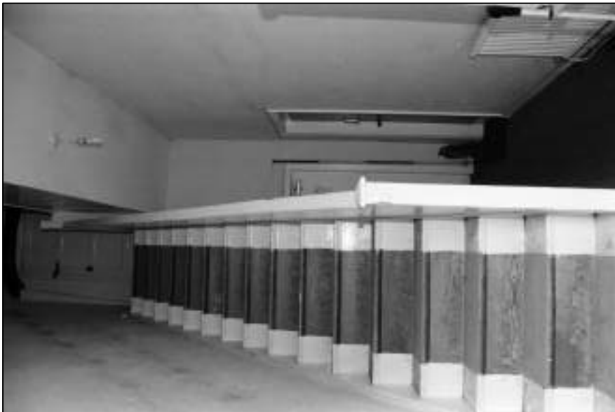
Appendix 2.24: General view of Building 3.2, room G11
