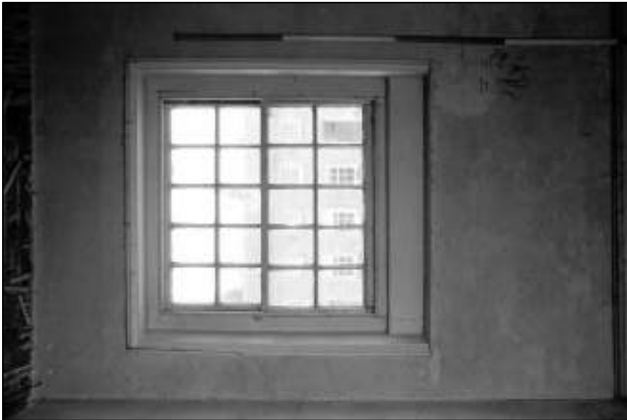
Appendix 2.87: Detail of window in Room F6 Building 3.3
