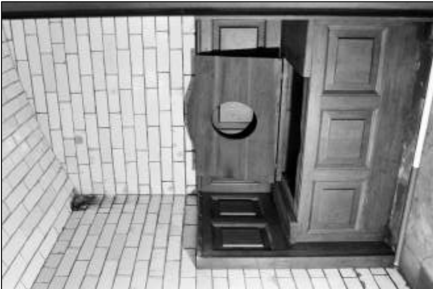
Appendix 2.153: General view of the southern room of Building 9.1
