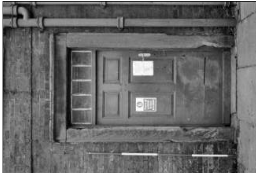
Appendix 2.48: Detail of door in north elevation of Building 3.3 , leading to room G8
