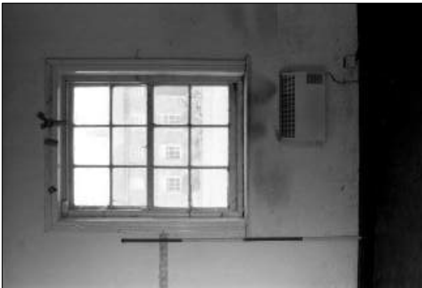
Appendix 2.61: Detail of window in north wall of Room G4 Building 3.3
