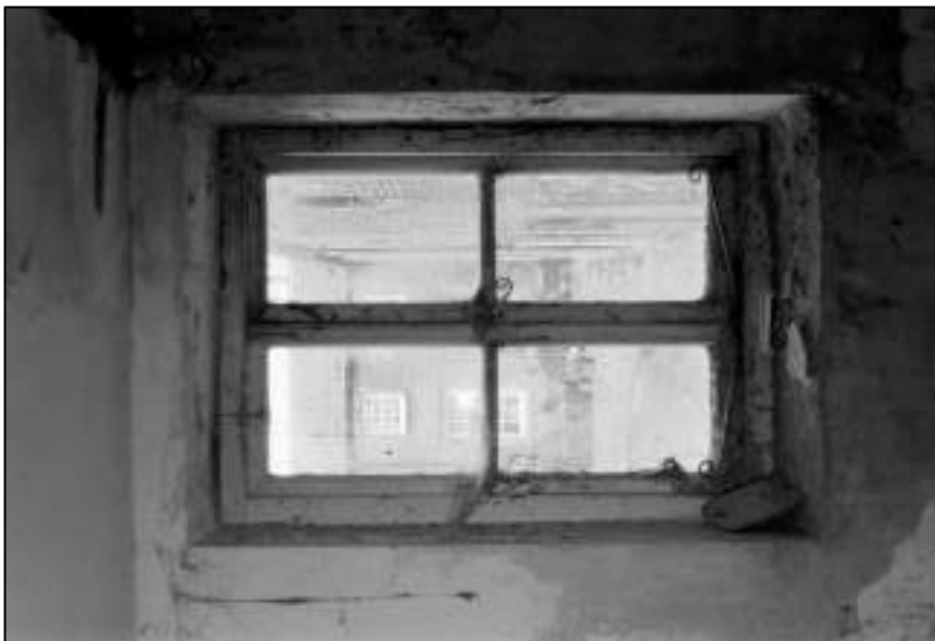
Appendix 2.86: Detail of window in Room F1 Building 3.3
