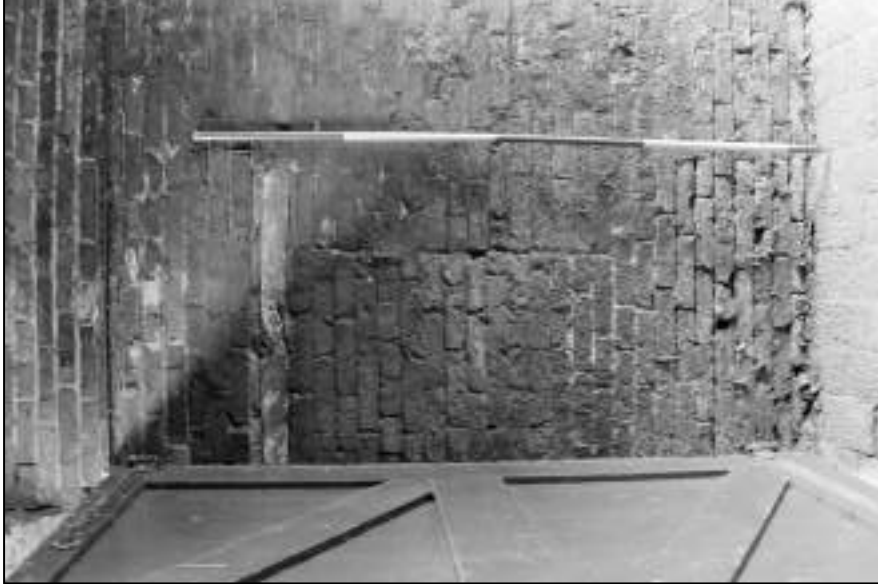
Appendix 2.77: Detail of blocking in the east wall of the Cart Passage, Building 3.3
