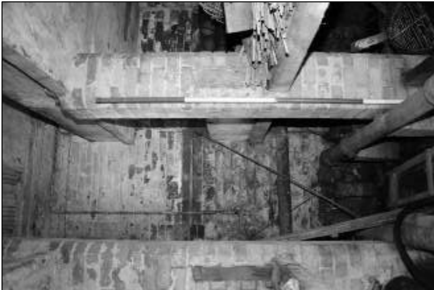
Appendix 2.136: General view of Room G3 Building 5.3
