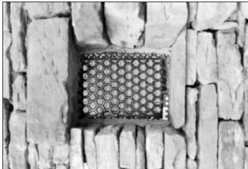
Appendix 2.152: Detail of vent in east elevation of Building 9.1
