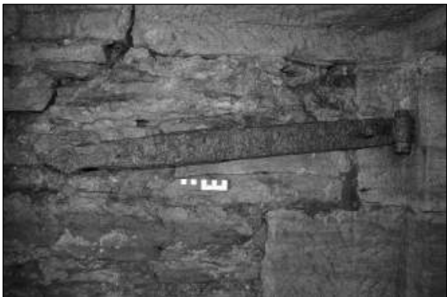
Appendix 2.158: Detail of strap hinge for removed door at edge of the ice pit in Building 9.2 , looking east
