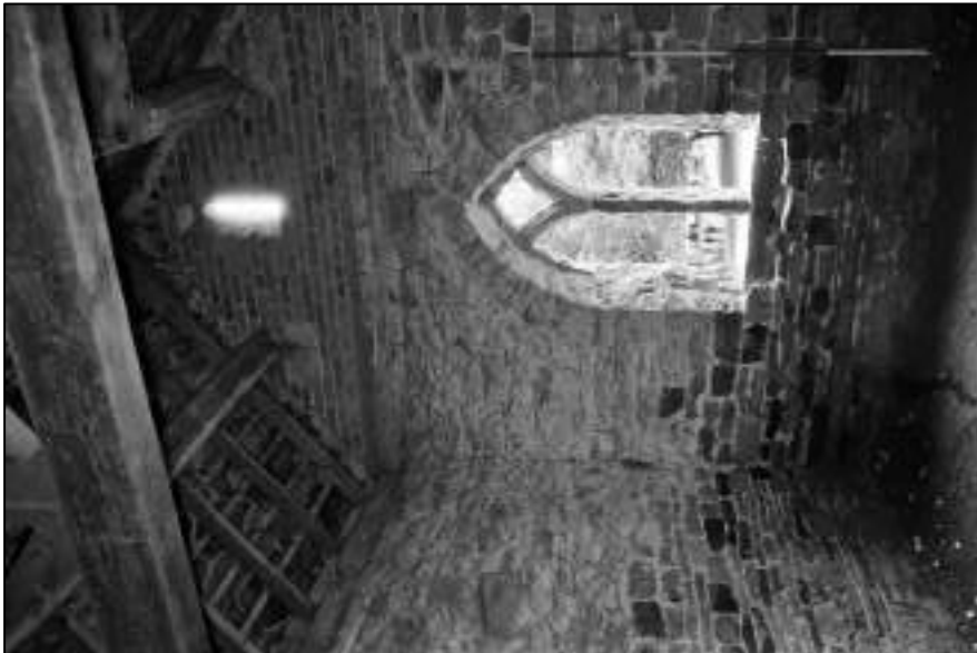
Appendix 2.165: General view of the eastern room of Building 12.1
