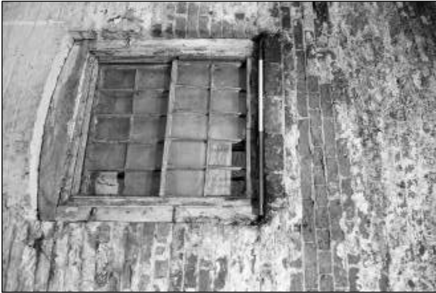
Appendix 2.137: Detail of window in east wall of Room G1 Building 5.3
