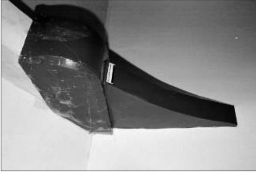
Appendix 2.35: Detail of corbel for truss in Building 3.2, room F13 (10cm scale; film 11.36)
