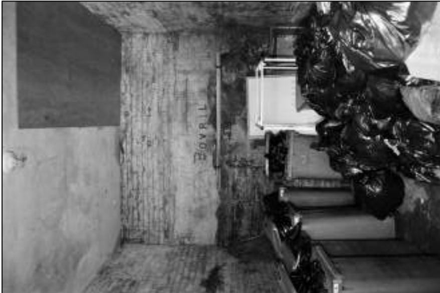
Appendix 2.76 General view of Room G8 Building 3.3
