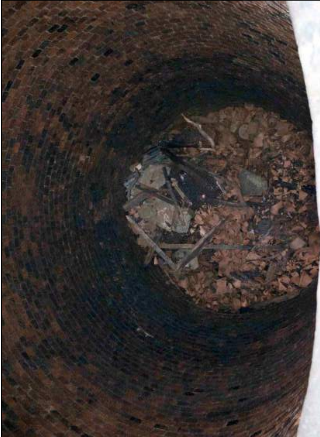
Appendix 2.159: General view of interior of the ice house, Building 9.2 , looking down (digital)
