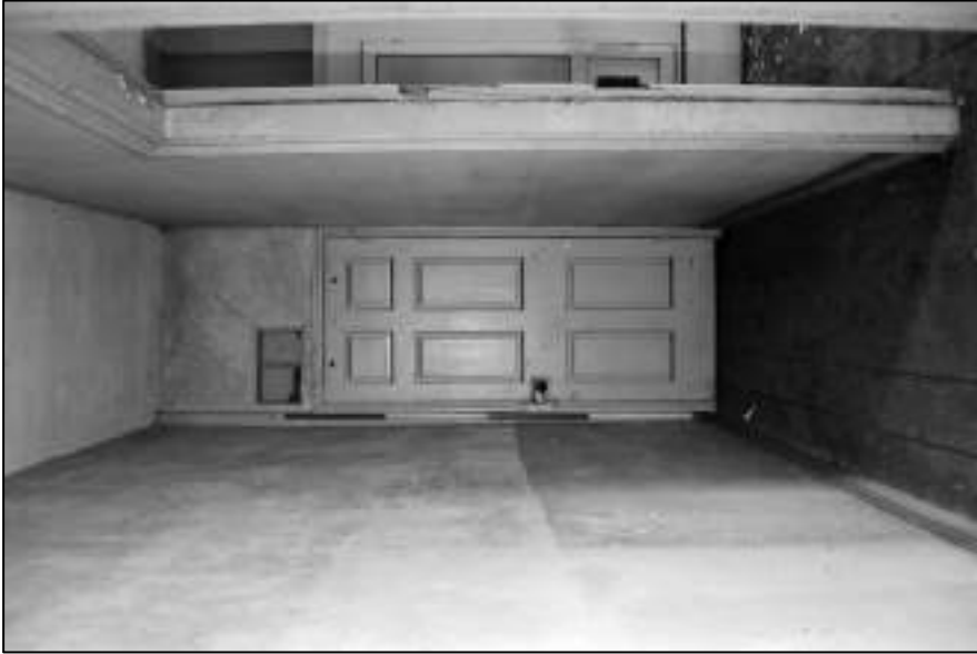
Appendix 2.85: General view of Room F5 Building 3.3
