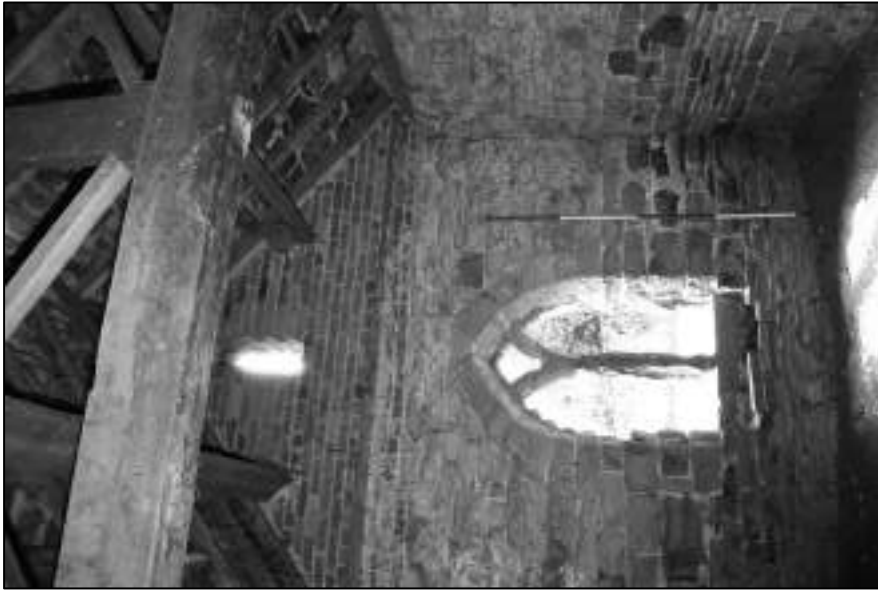
Appendix 2.166: General view of the western room of Building 12.1
