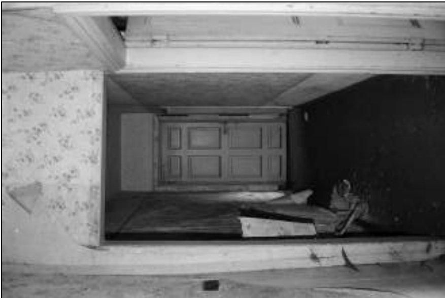
Appendix 2.93: General view of Room F10 Building 3.3
