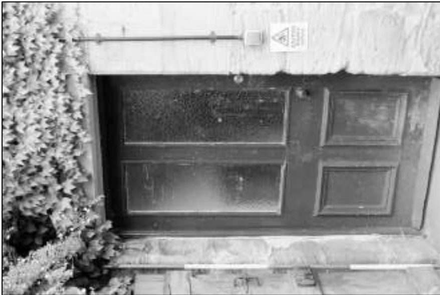
Appendix 2.17: Detail of door in south elevation of Building 3.2
