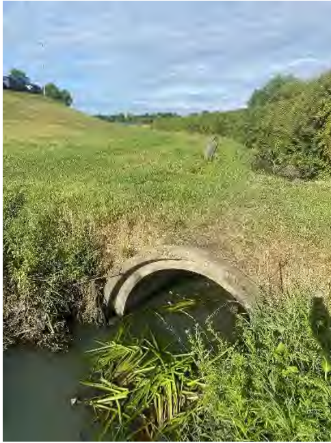
Figure 12. TRIB_004 upstream inlet- 1.35m diameter culvert
