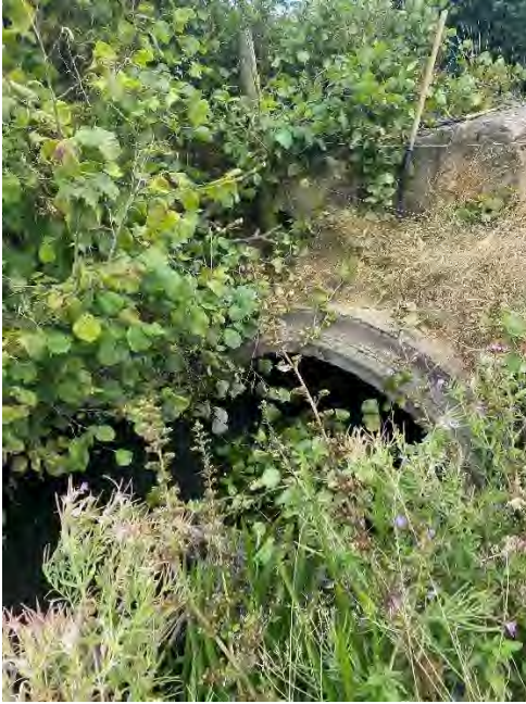
Figure 13. TRIB_007 downstream outlet - 1.75m diameter culvert
