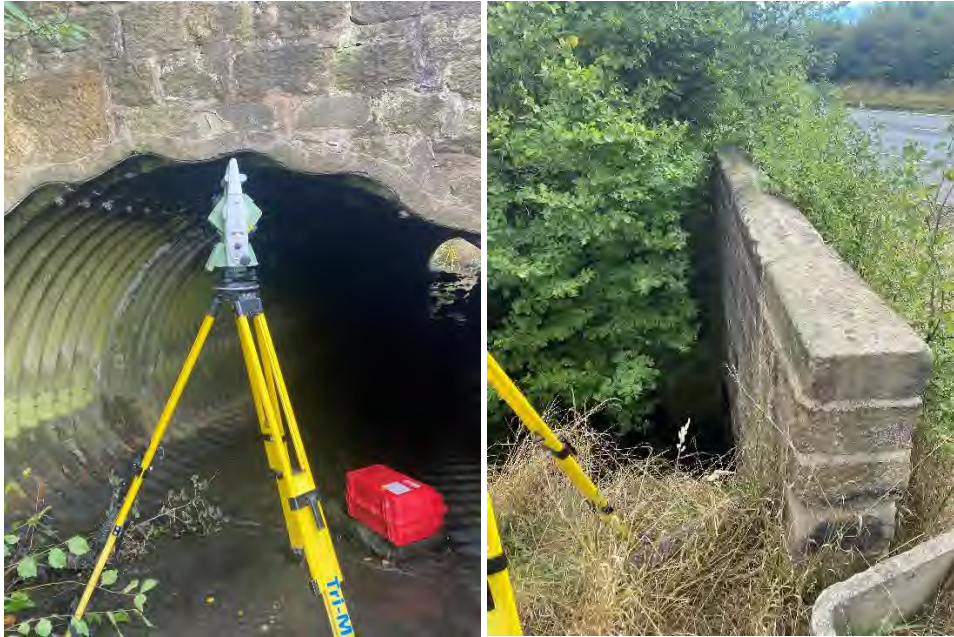
Figure 10. CARR_007 upstream inlet - A635 Culvert
