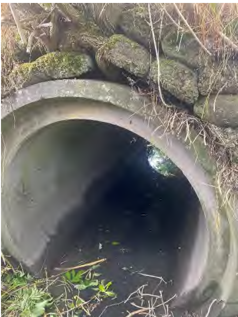
Figure 14. TRIB_011 upstream inlet - 1.5m diameter culvert
