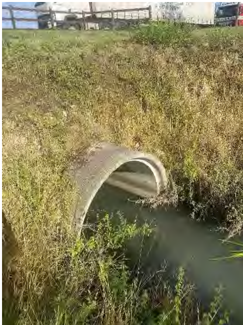
Figure 11. TRIB_002 upstream inlet- 1.9m diameter culvert
