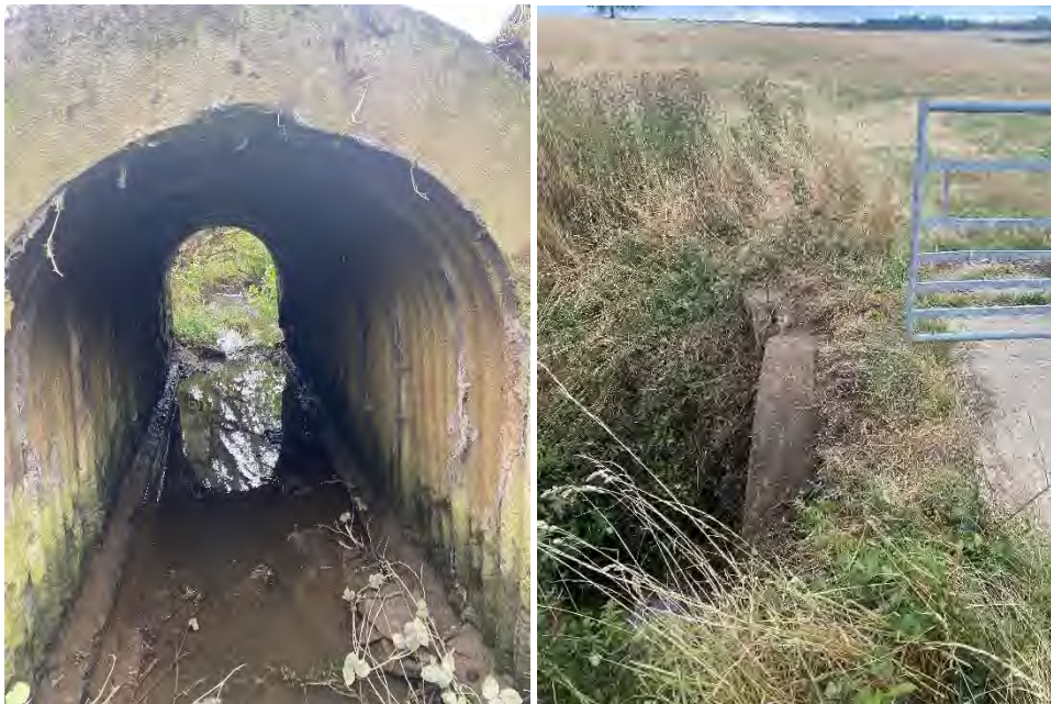
Figure 9. CARR_002 upstream inlet - Farm Access Culvert
