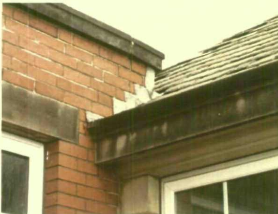
Figure 3: loose flashing to south of Maths & Geography (1930's buildings)
