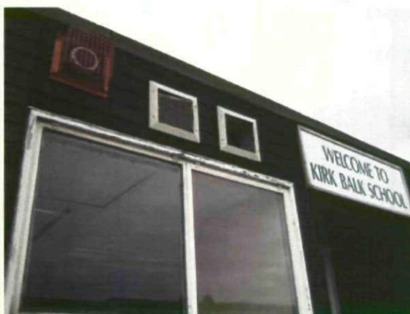
Figure 6: missing grills on vents, giving access to roof space in science block
