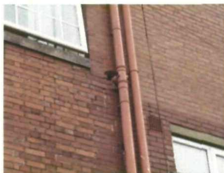
Figure 2: Rear building (B-block), hole in brickwork
