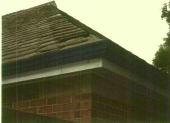
Figure 3: loose flashing to south of Maths & Geography (1930's buildings)
