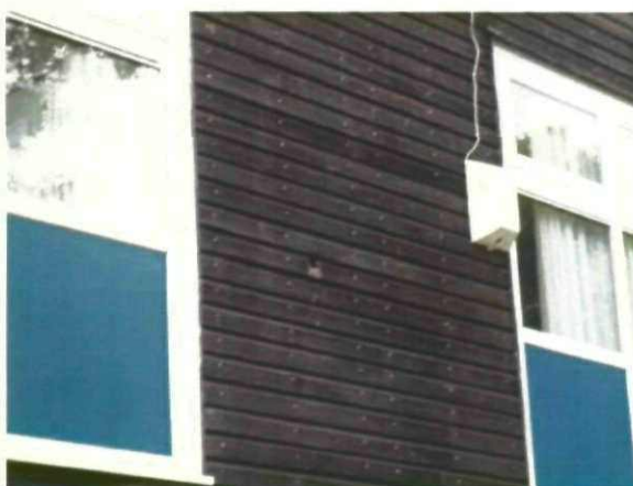
Figure 6: missing grills on vents, giving access to roof space in science block
