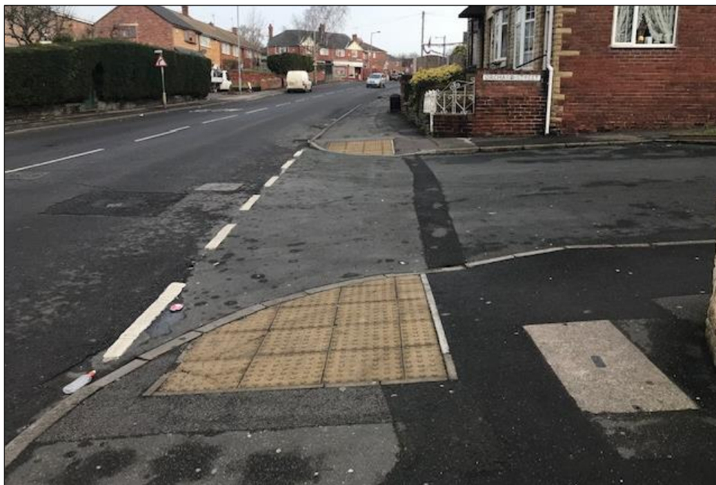
Figure 8. Dropped Kerbs and Tactile Paving North of B6098 Goldthorpe Road
