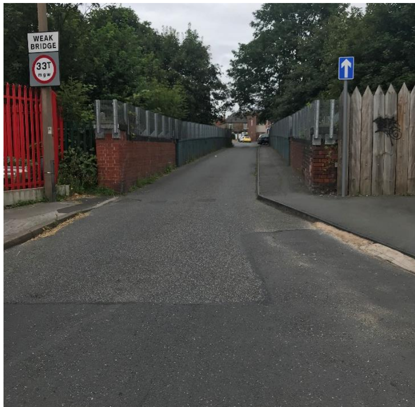
Figure 6. Straight Lane open to Vehicular Traffic
