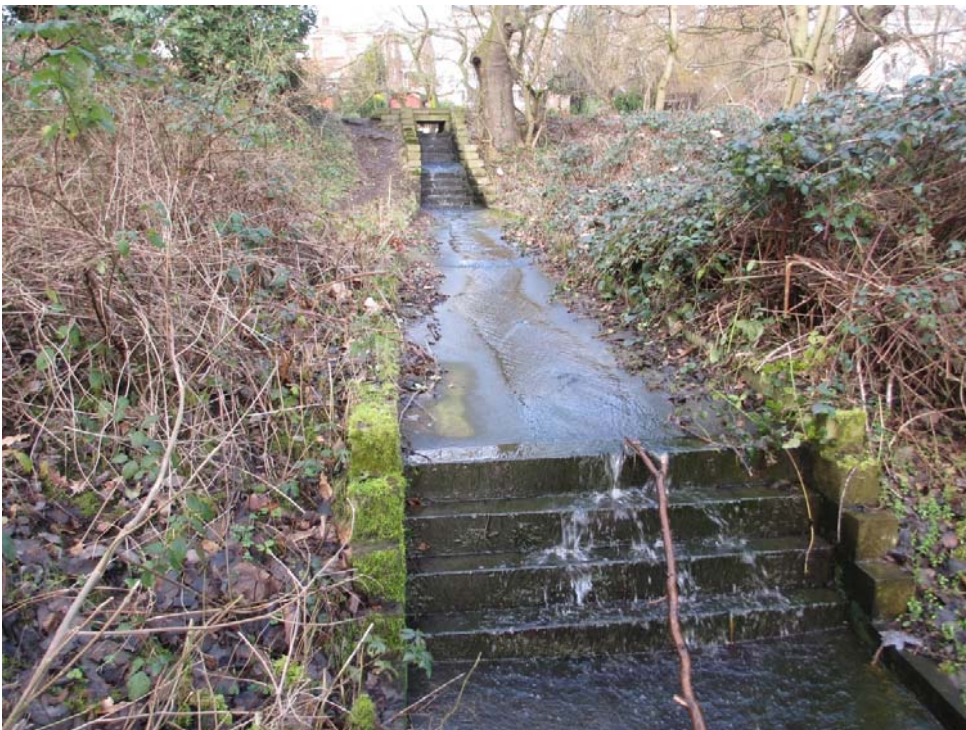
Spillway from Overflow
