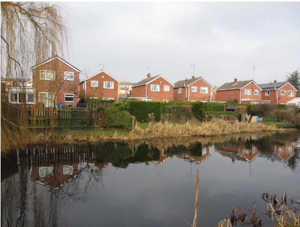
Properties east of site with gardens adjacent to canal at risk of flooding
