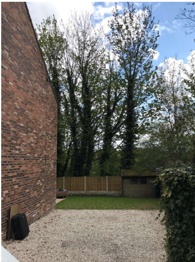
Fig 04. Space for extension to south side of existing dwelling.
