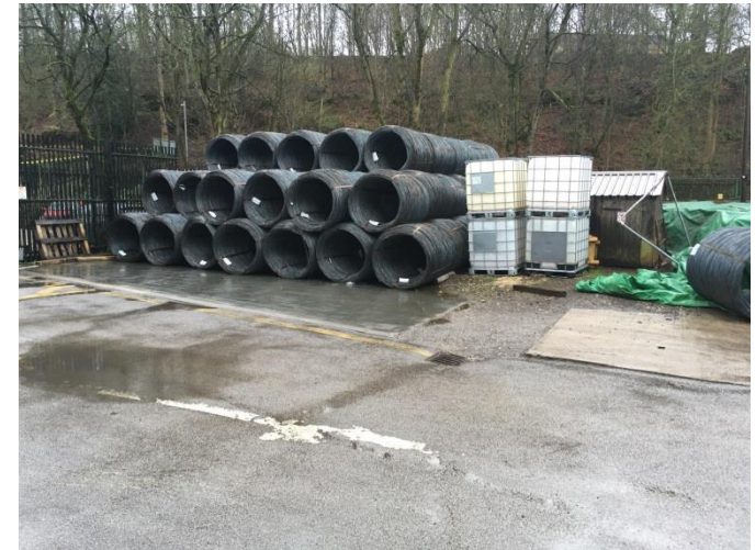
The site now this building has been demolished
