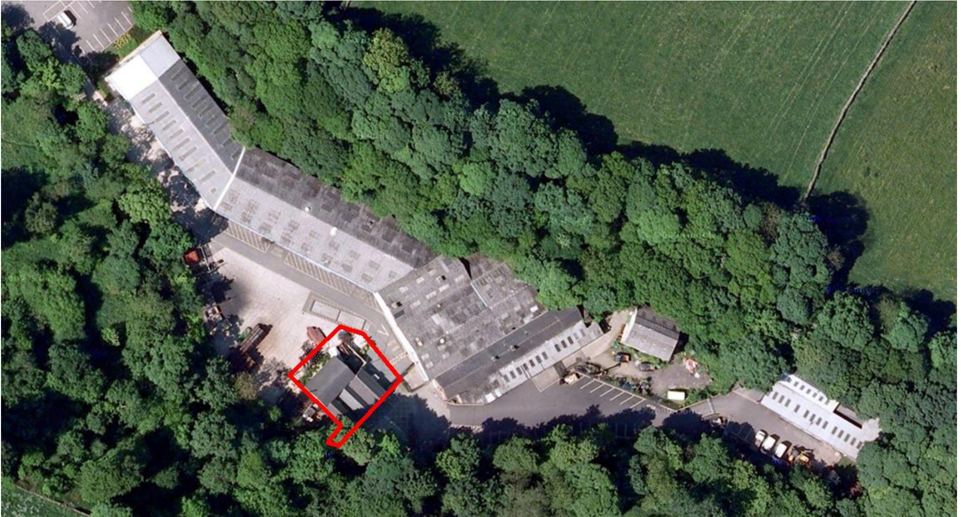
Construction of Office Building
