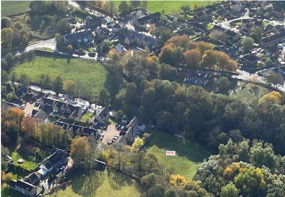
Fig 01. Aerial Photo showing proposed development site.
