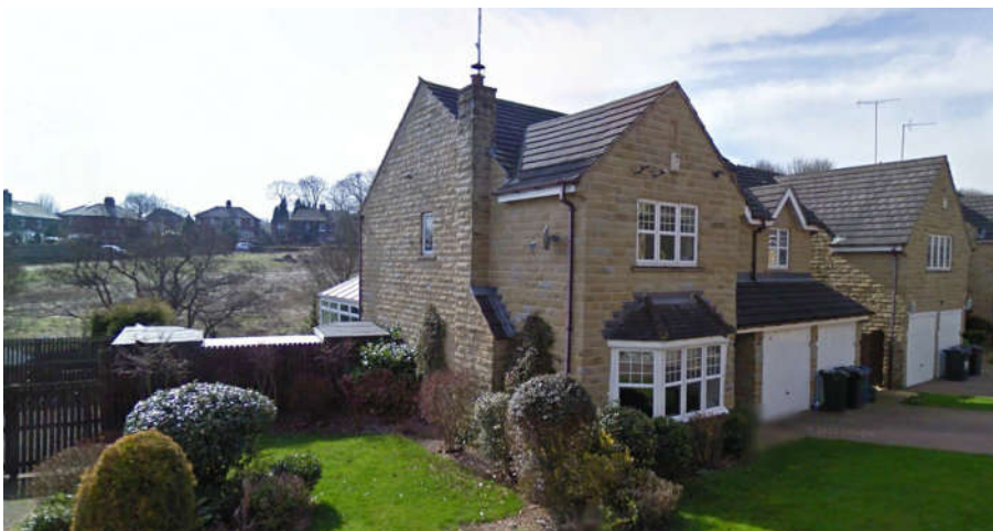
Fig 09. Example of existing housing to Millstones.
