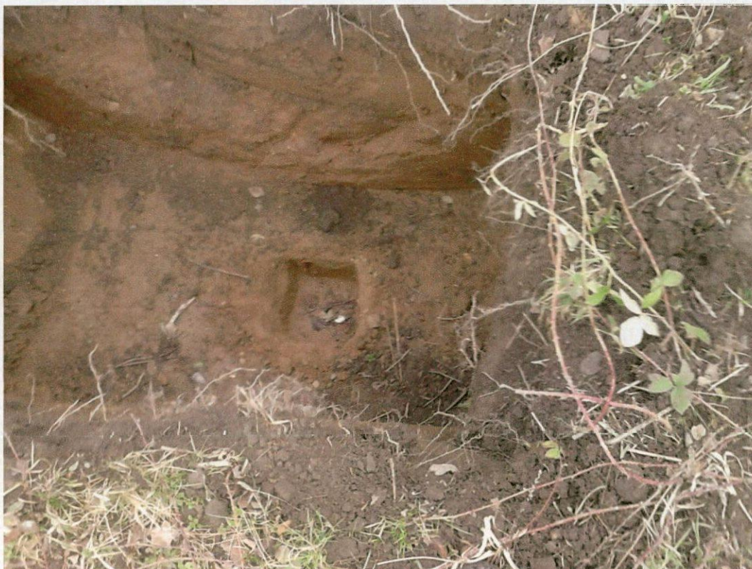
Photograph 4 –Trial Hole 06/02/2017 after rainfall
