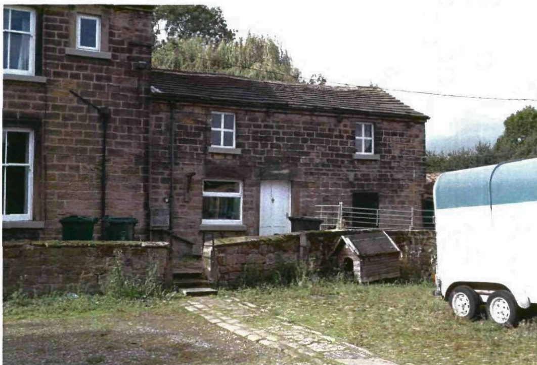
10B The north east elevation of the existing farm cottage
