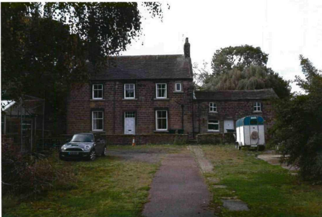
10A The north east elevation of the farmhouse
