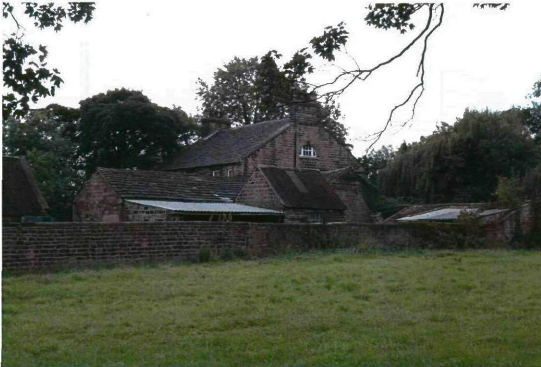
20. Existing house and farm buildings at Stud Farm taken from the adjoining field
