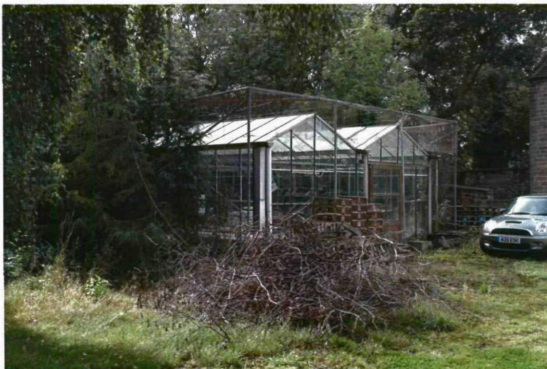
13. Existing glasshouses and outbuildings to the south east of the farmhouse
