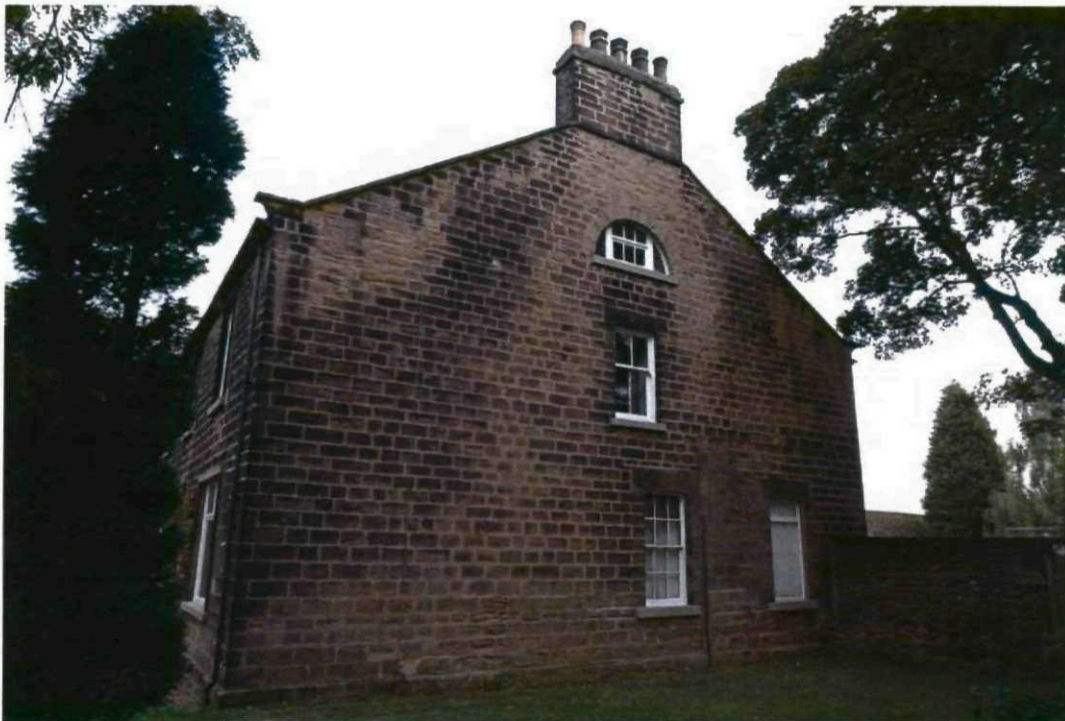
16. South gable elevation of the farmhouse
