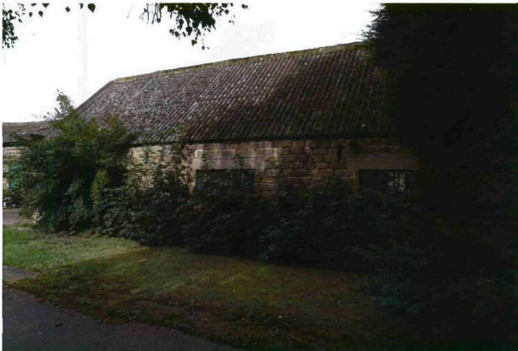
12. The south east elevation of single storey barn adjoining Church Street
