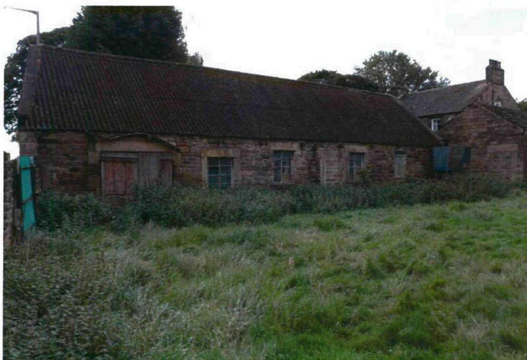
18. The north elevation of the existing single storey stone barn adjoining Church Street
