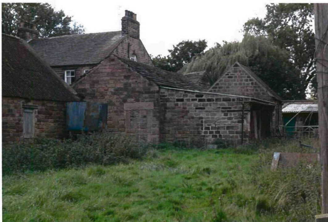
19. Single storey stone barn and outbuildings at the north side of the existing farm courtyard
