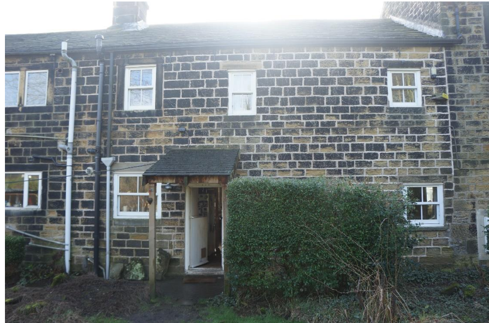
7 Ingbirworth Road Photo - Rear
