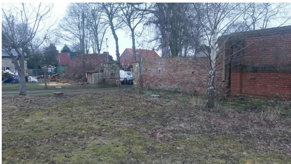
Fig 2 Existing north boundary wall and gates
