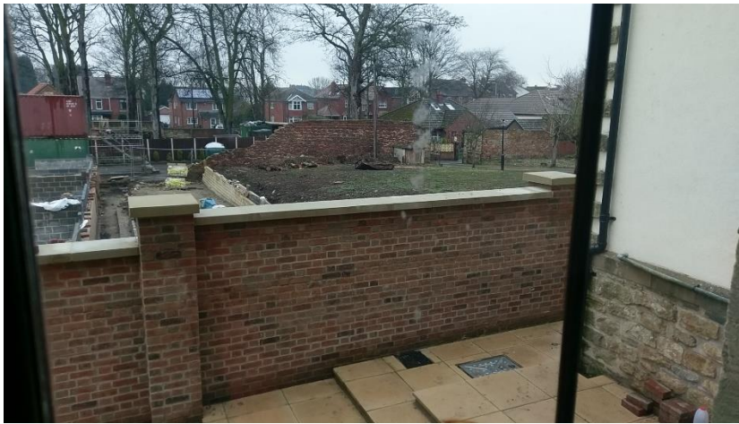
Fig 3 New brick wall with piers and PC copings
