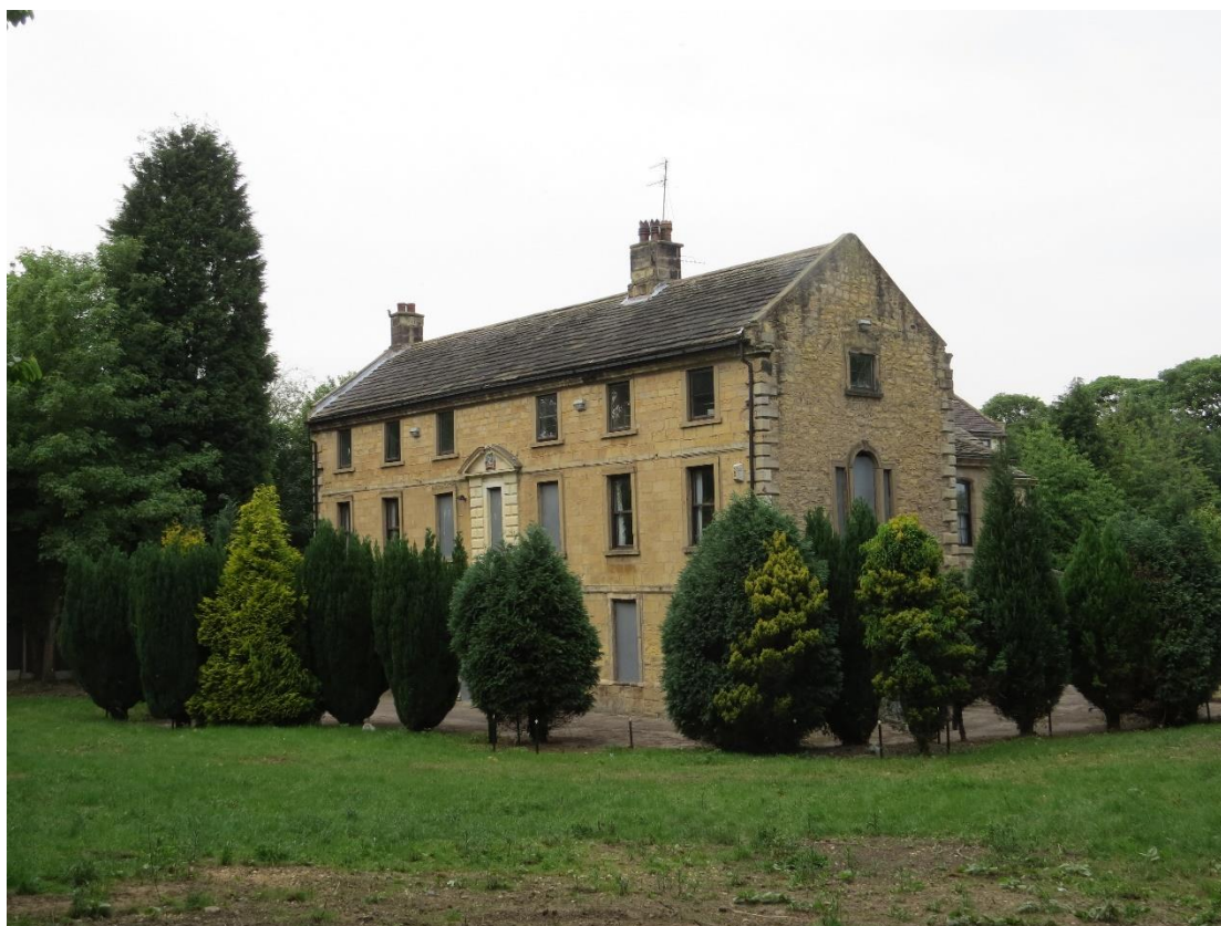
Fig 1. View of south elevation
