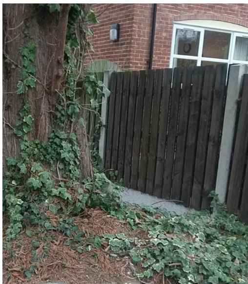
Fig 4 Vertical boarded fence with concrete posts and base rail
