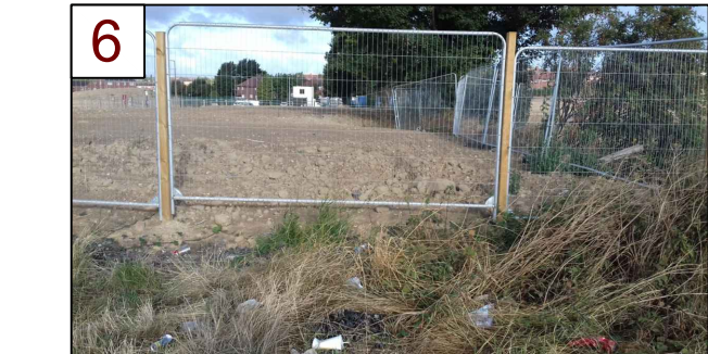
View west into additional site area
