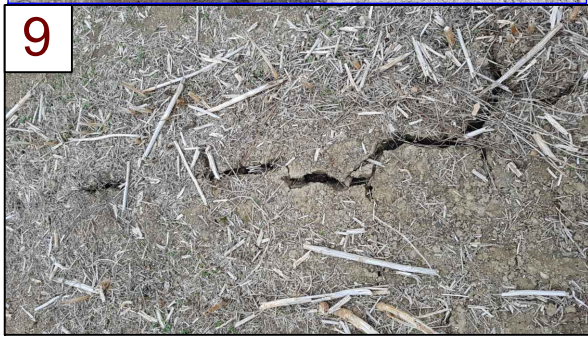
Example of dried and cracked soils
