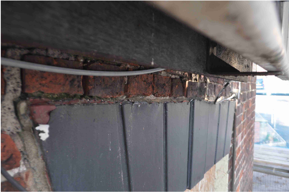
Figure 34: Photo 28. Detail showing top of lintel.
