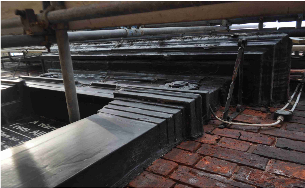
Figure 25: Photo 18. Anta, capital, frieze and architrave close up from underneath.
