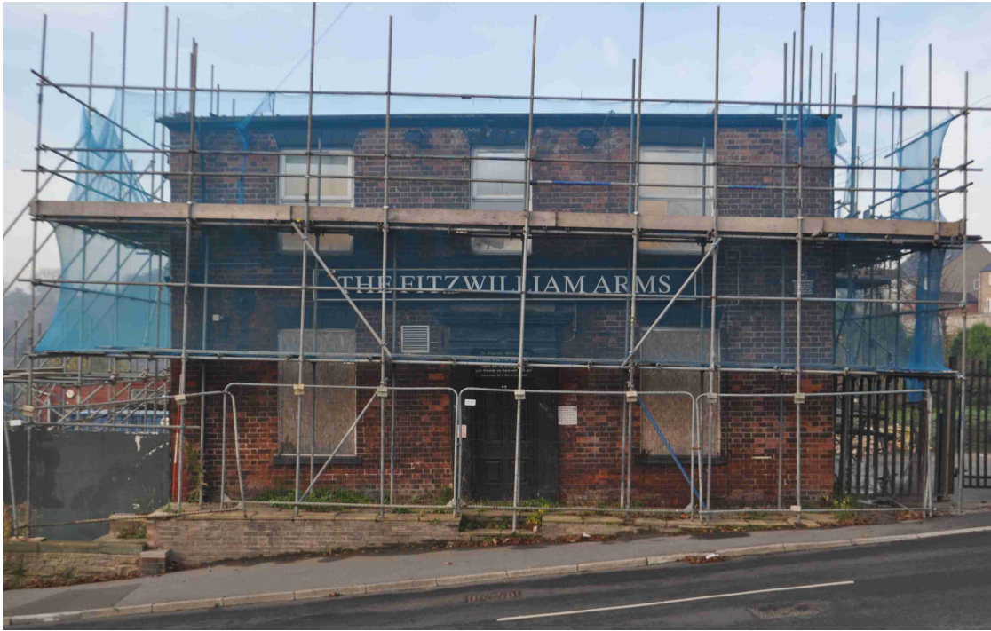
Figure 11: Photo 4. Northeast facing elevation.
