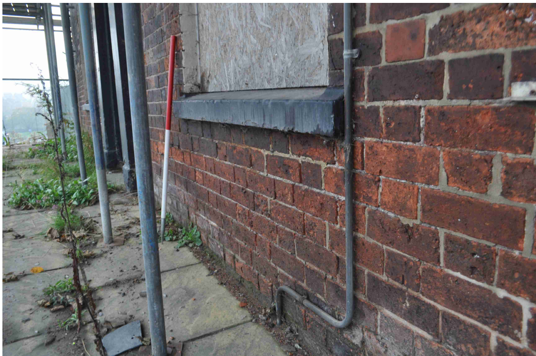
Figure 18: Photo 11. Window sill.
