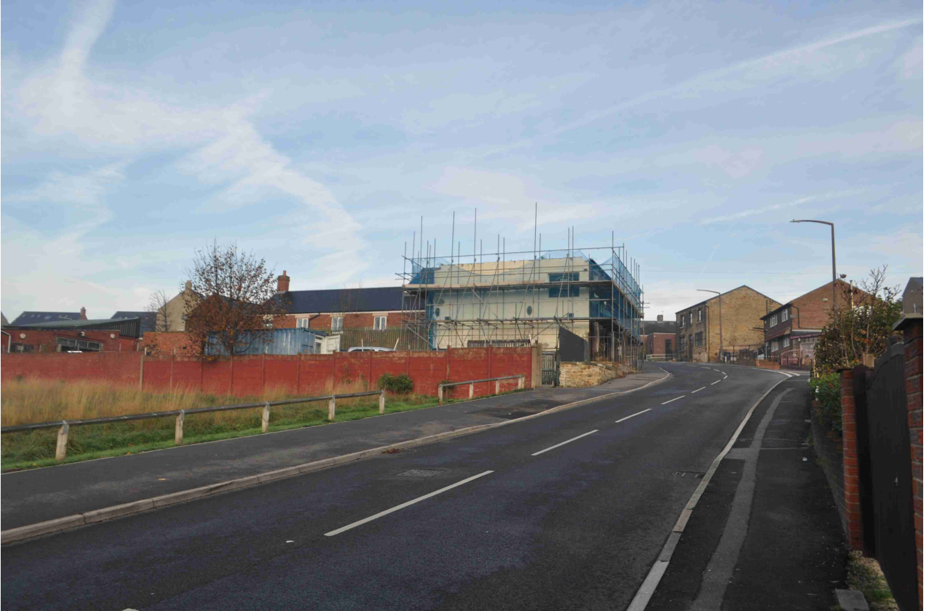
Figure 8: Photo 1. Landscape setting from downslope
