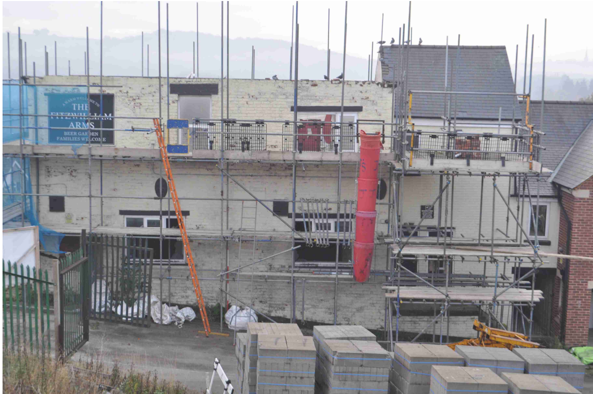
Figure 15: Photo 8. Northwest facing elevation.
