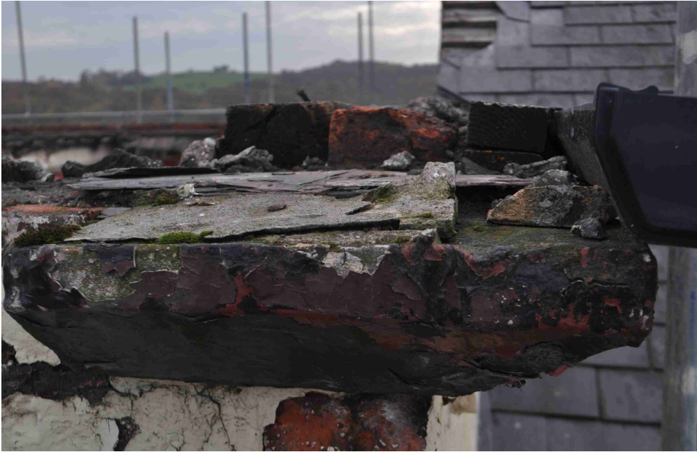
Figure 50: Photo 44. Northeast end of architrave surmounting southwest facing wall.
