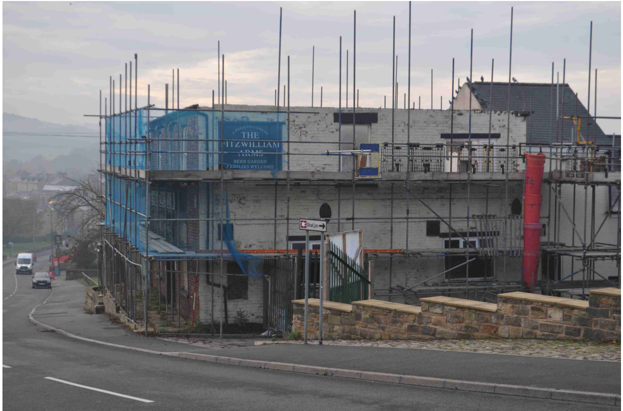
Figure 13: Photo 6. Northeast and northwest facing elevations.
