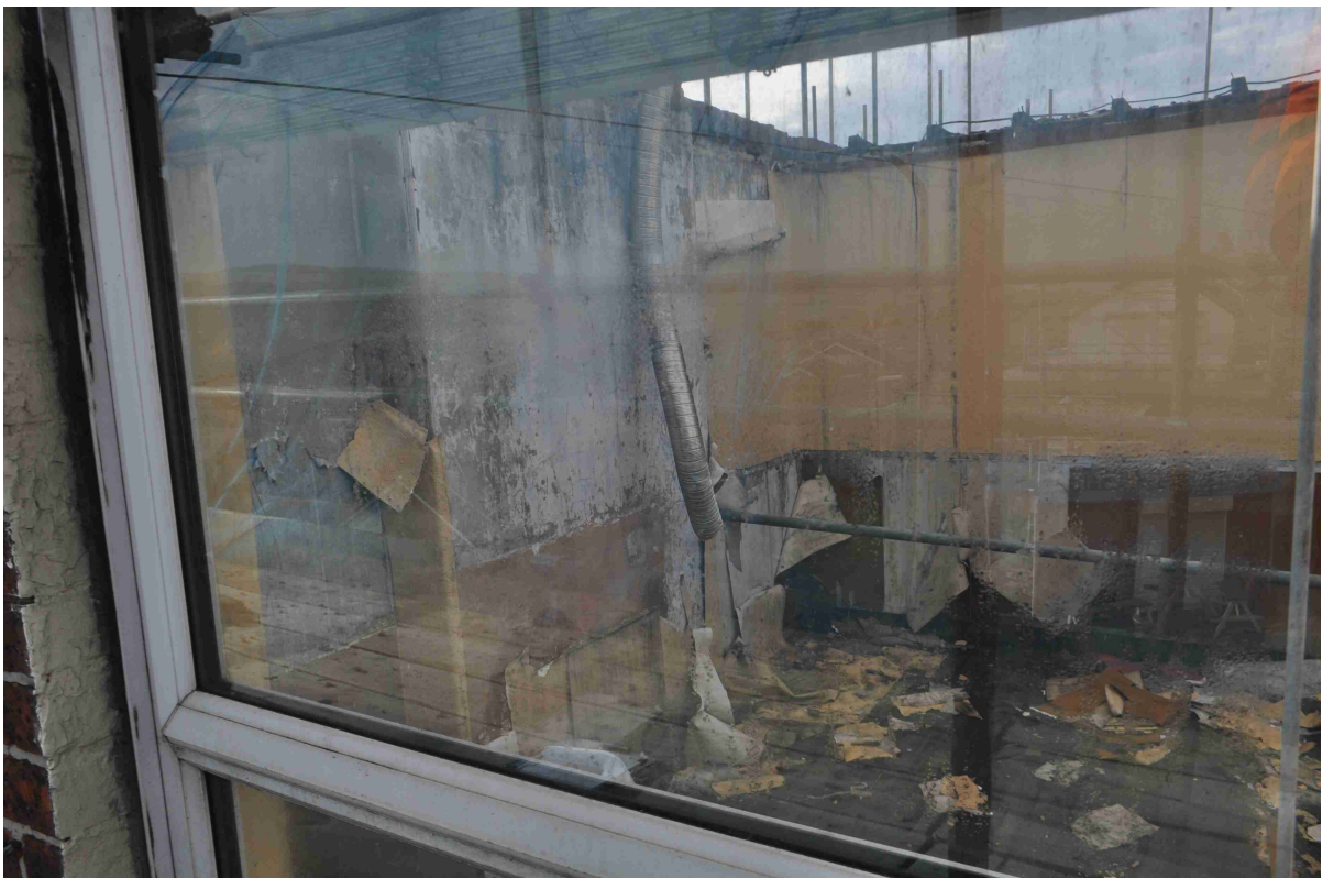
Figure 62: Photo 56. Interior, featuring chimney breast.
