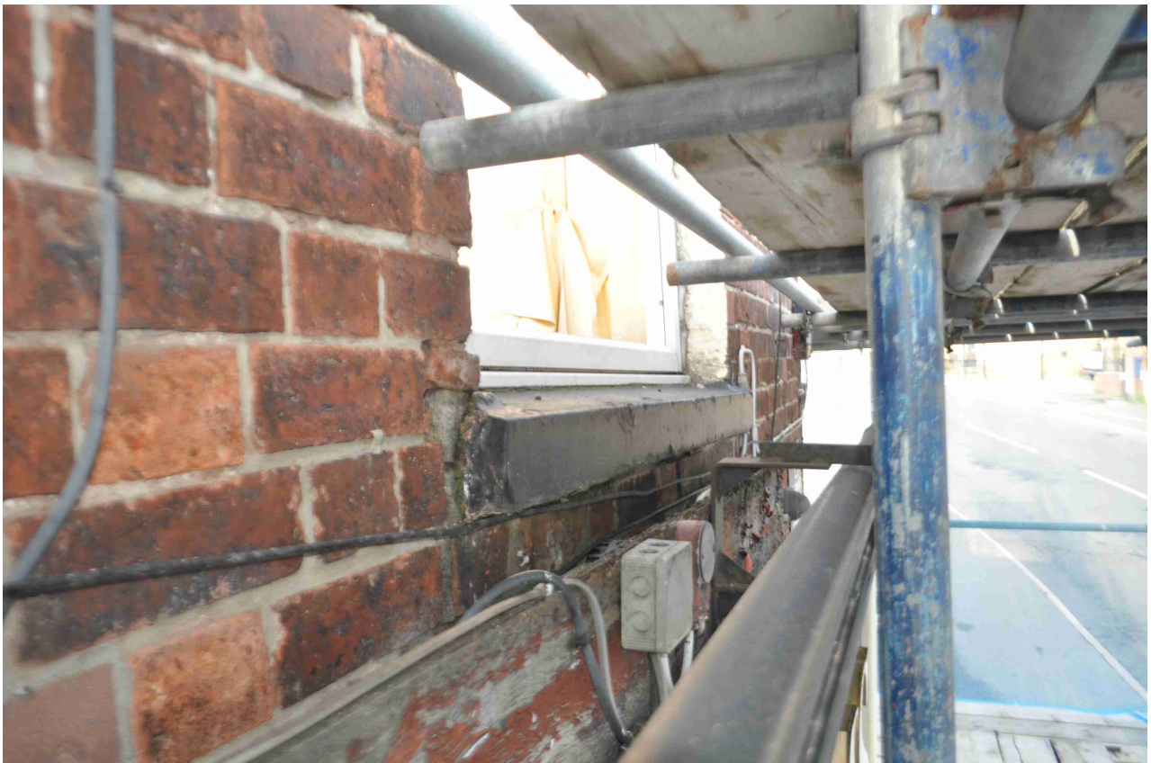
Figure 43: Photo 37. Window sill.
