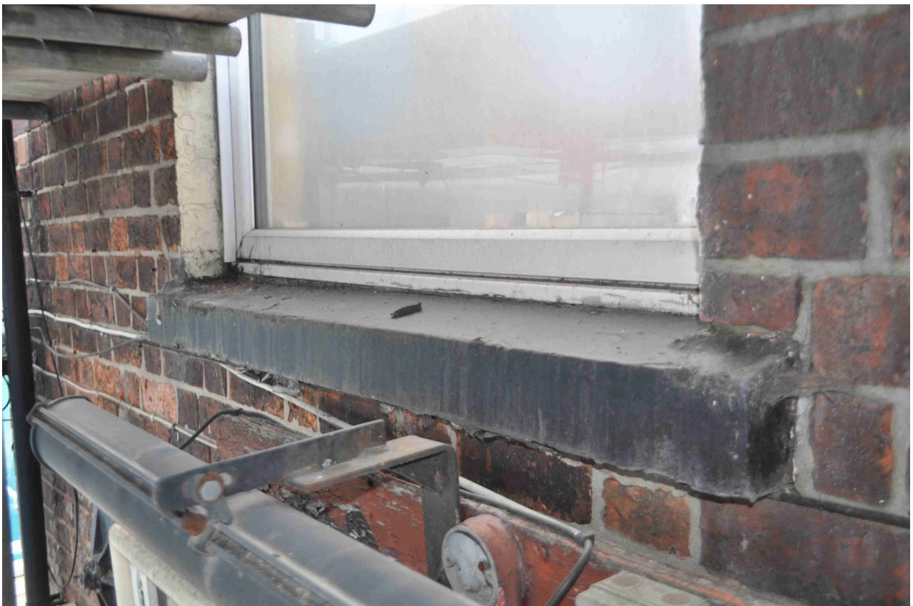
Figure 47: Photo 41. Window sill.
