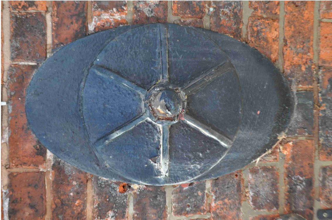
Figure 38: Photo 32. Wall tie.
