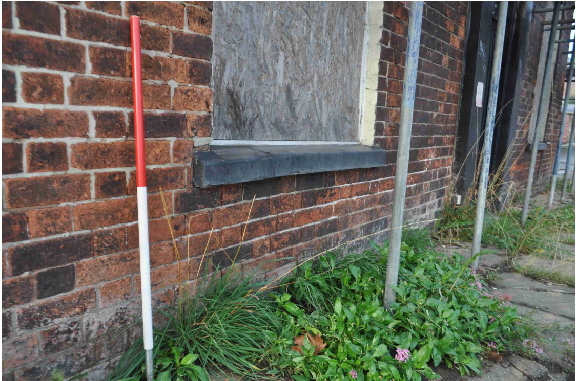
Figure 19: Photo 12. Window sill.
