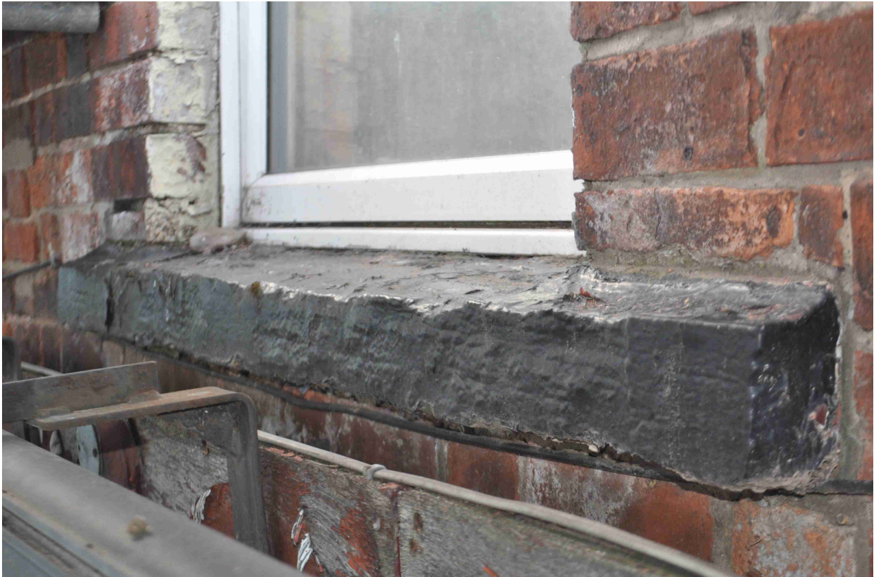
Figure 45: Photo 39. Window sill.
