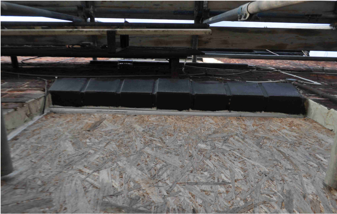
Figure 21: Photo 14. Lintel, from underneath.
