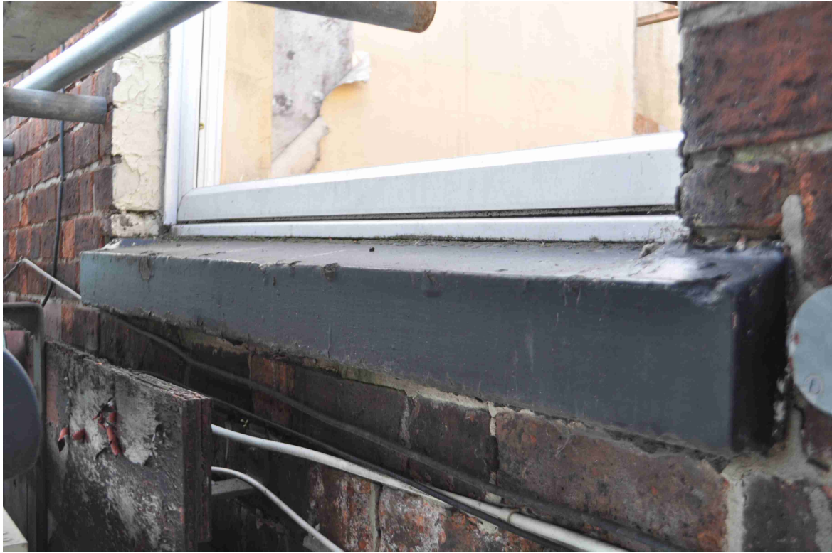
Figure 44: Photo 38. Window sill.
