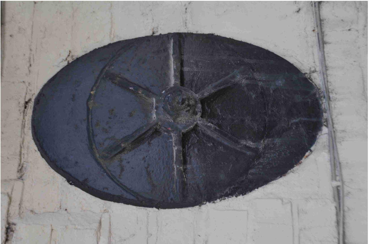
Figure 29: Photo 22. Wall tie.
