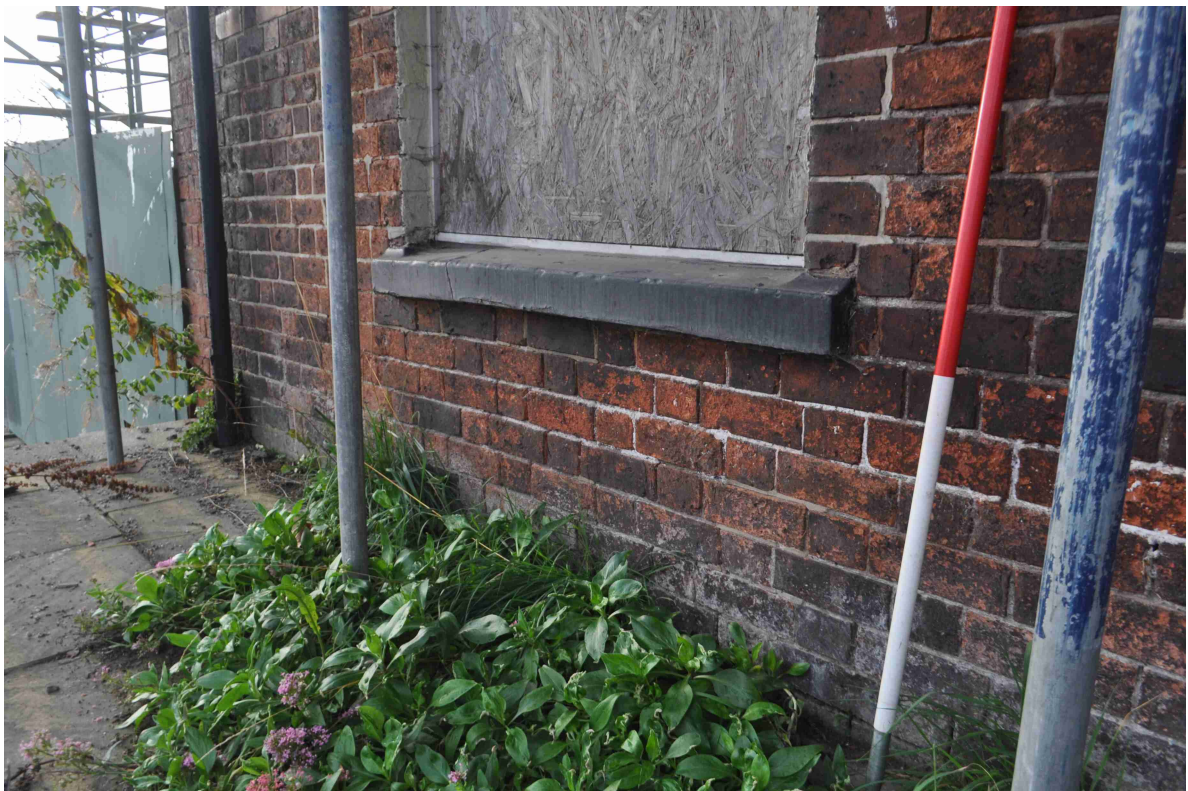
Figure 20: Photo 13. Window sill.
