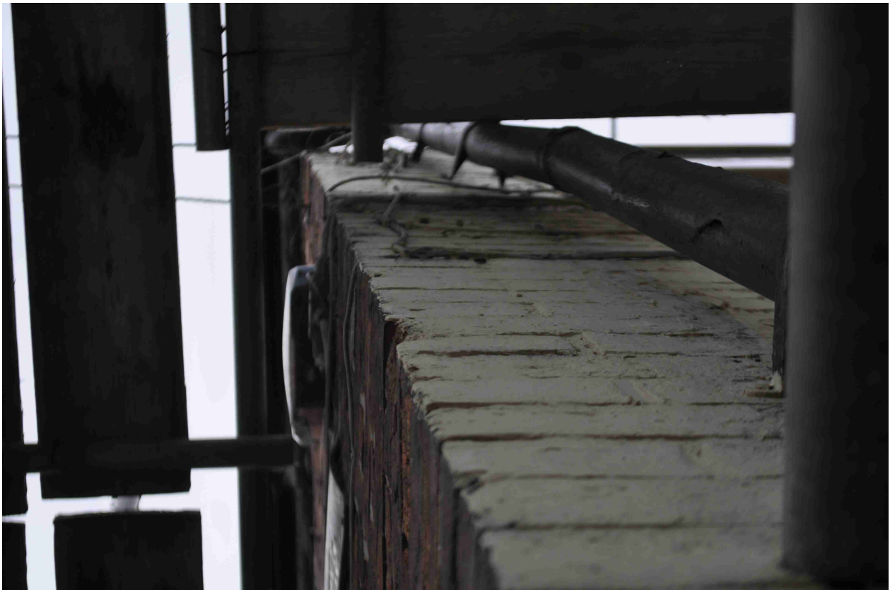
Figure 16: Photo 9. Downpipe and architrave at north corner.
