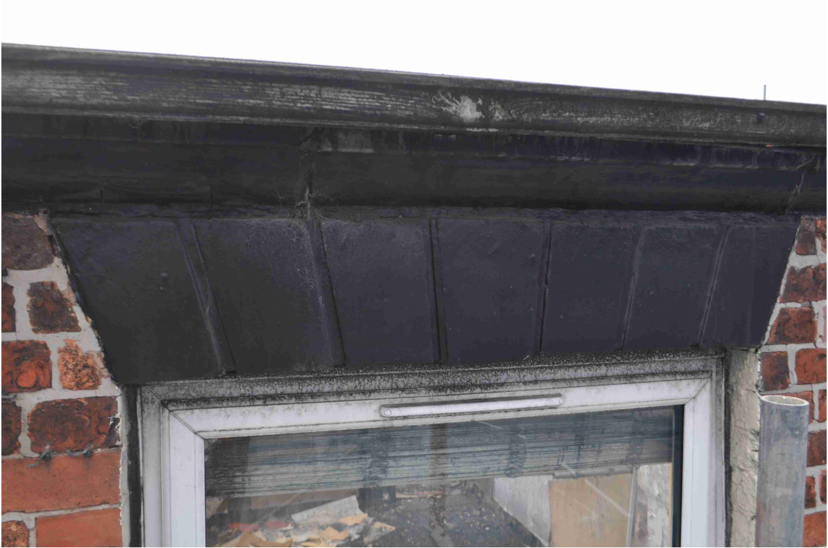
Figure 58: Photo 52. Lintel, architrave and gutter.
