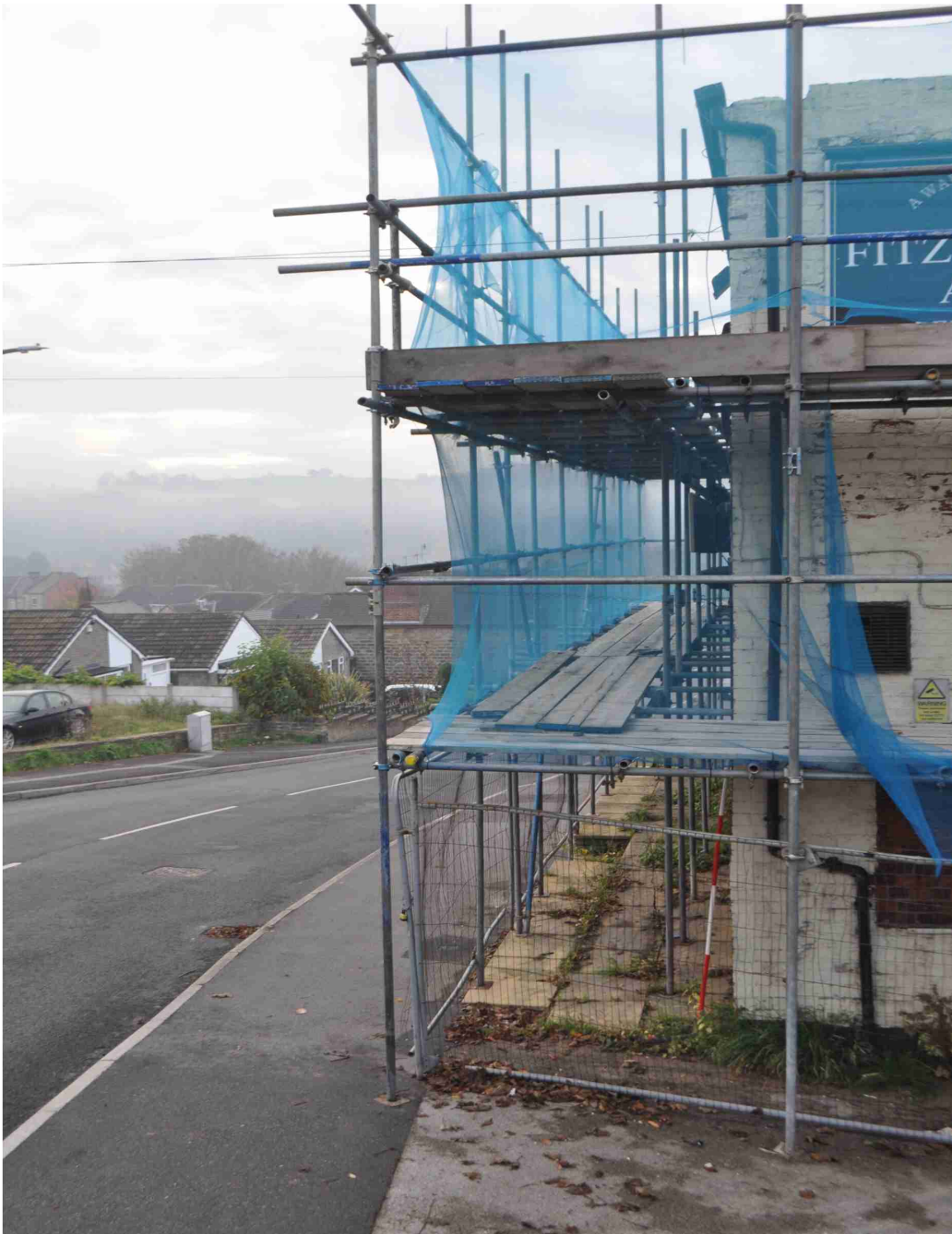
Figure 14: Photo 7. North corner showing downpipe and gutter.
