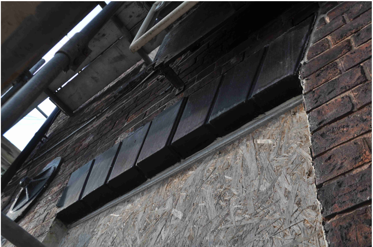
Figure 22: Photo 15. Lintel, from underneath.
