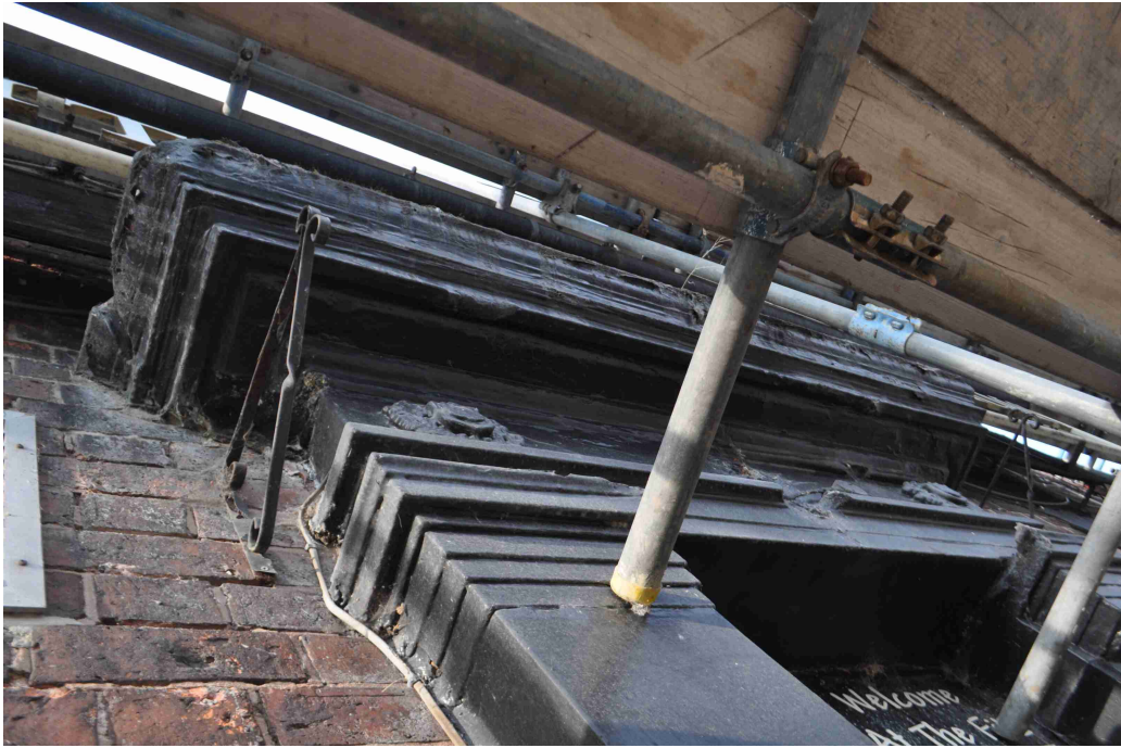
Figure 24: Photo 17. Anta, capital, frieze and architrave from underneath.
