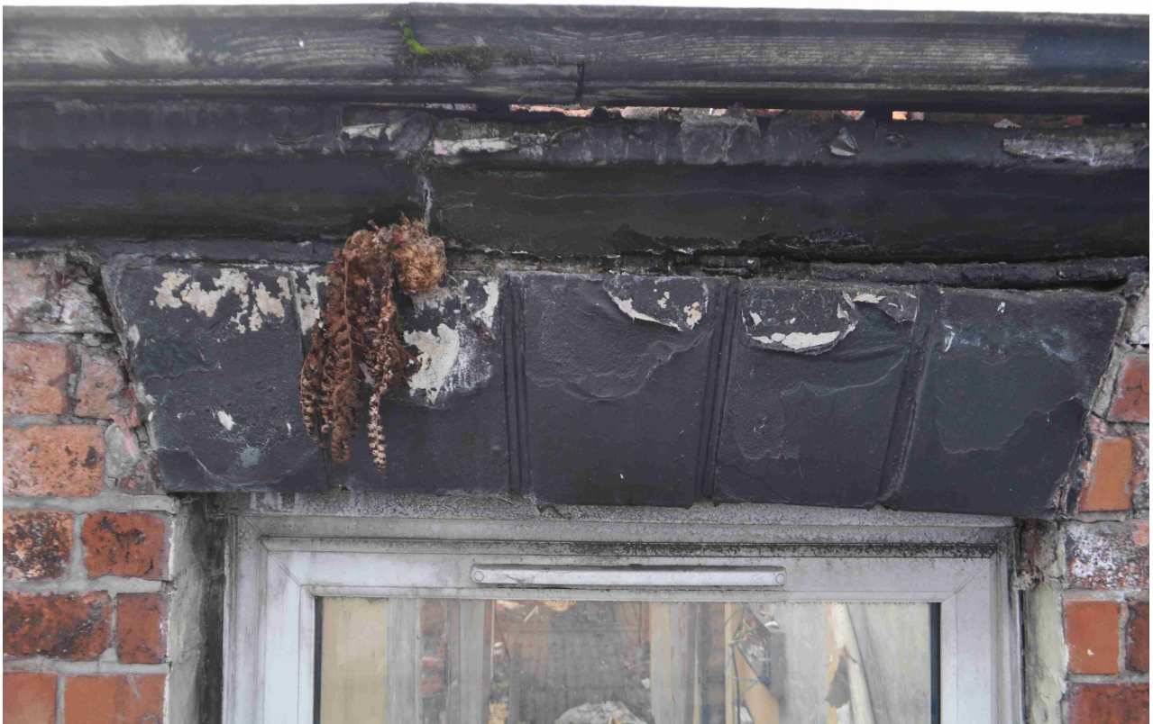
Figure 57: Photo 51. Lintel, architrave and gutter.
