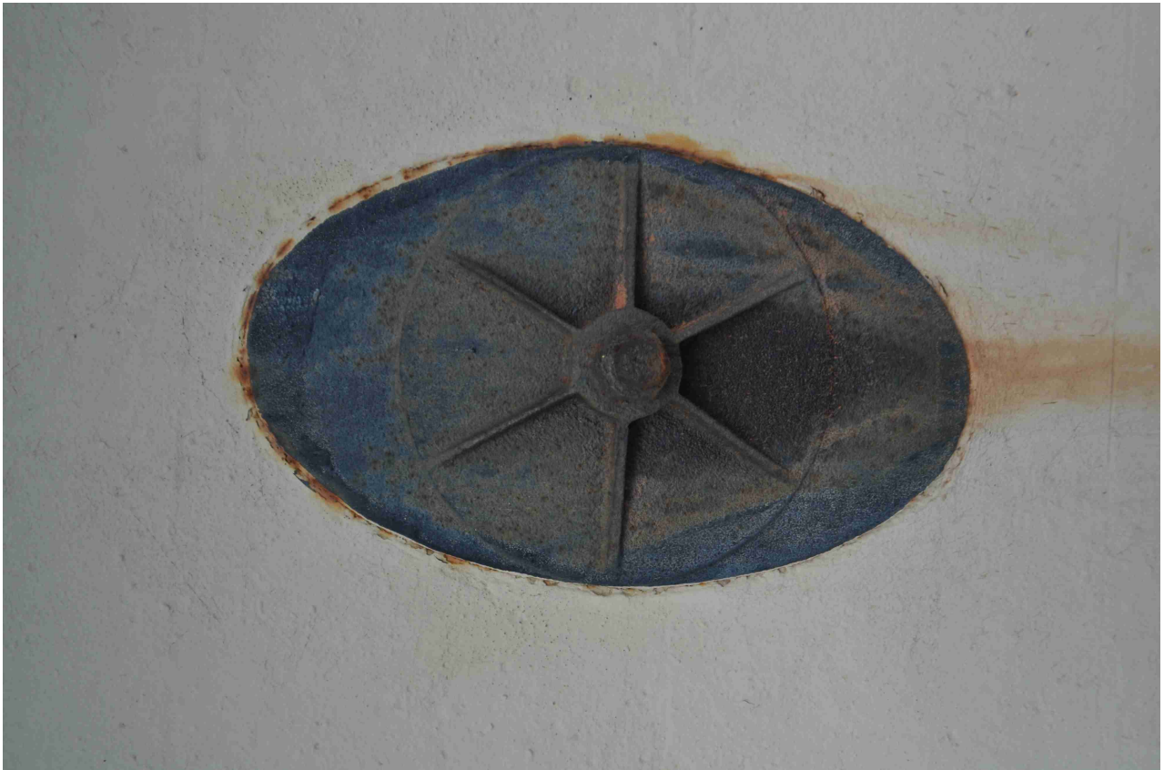
Figure 49: Photo 43. Wall tie.
