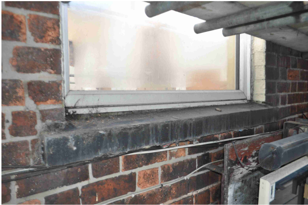
Figure 48: Photo 42. Window sill.
