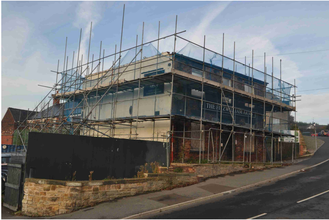
Figure 9: Photo 2. Northeast and southeast facing elevations
