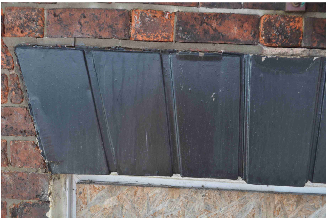
Figure 37: Photo 31. "Corbelled" lintel detail.
