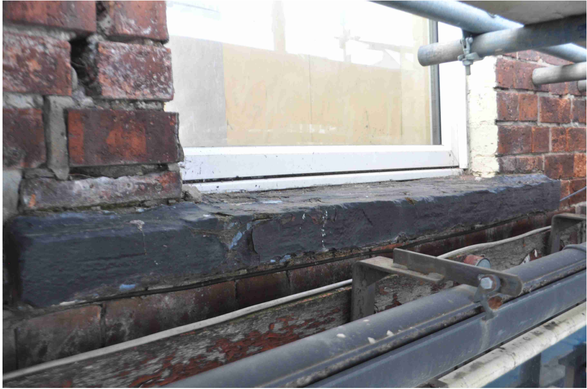
Figure 46: Photo 40. Window sill.
