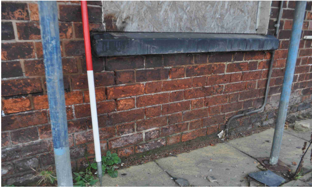
Figure 17: Photo 10. Window sill.
