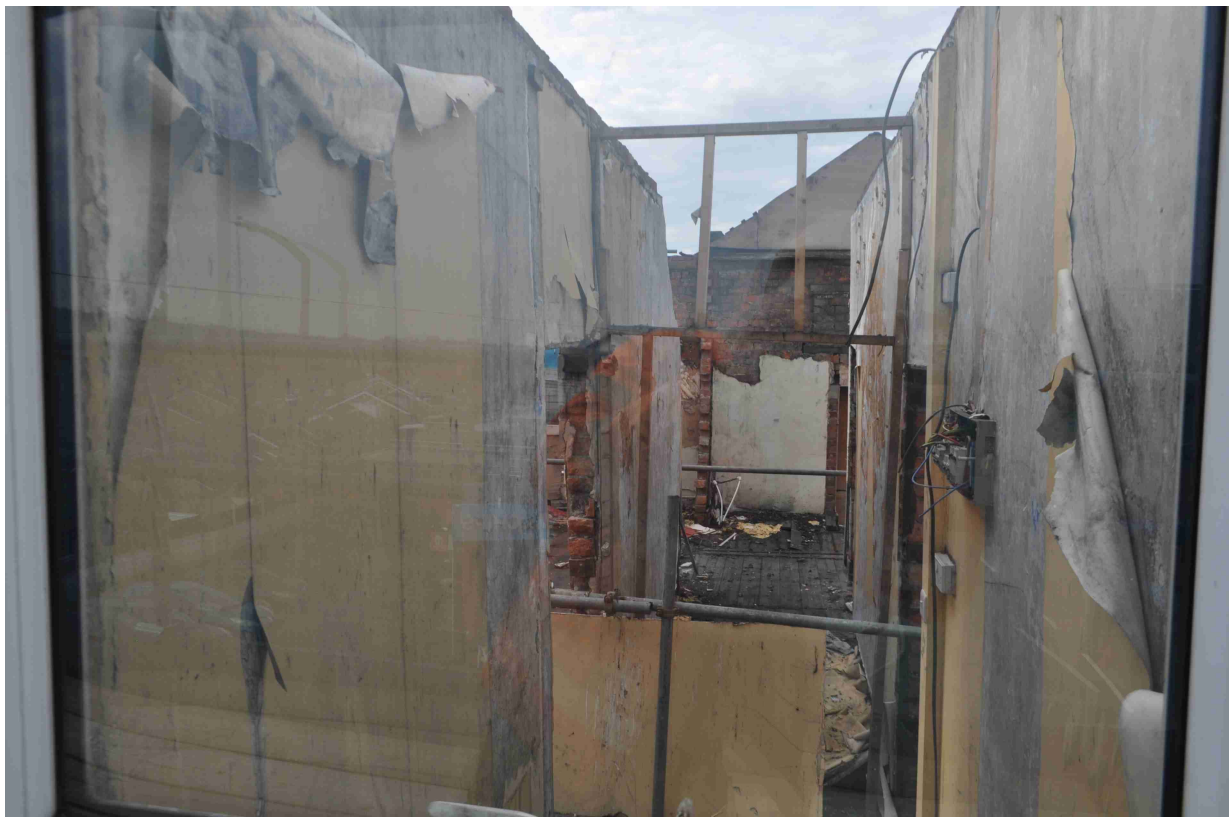
Figure 64: Photo 58. Interior corridor.
