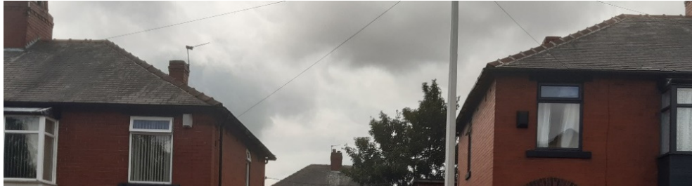
Above: Roofscape to No's 4 and 6 Overdale Avenue (Streetscene view)
