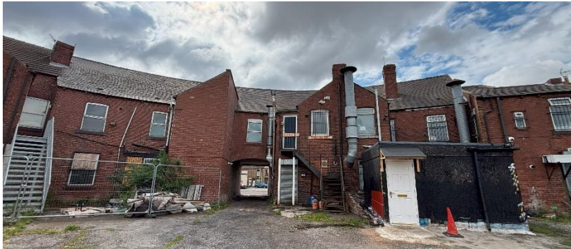
Figure 3 View of the back of the building from the northwest.
