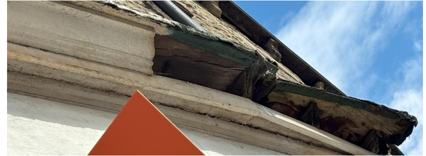
Figure 6 Showing large gap above of tunnel.
