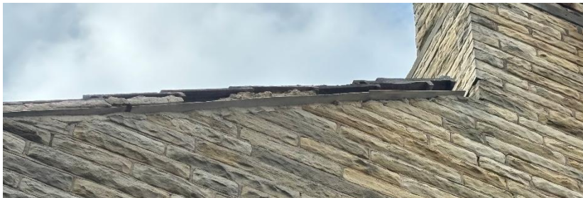
Figure 10 Showing gaps under the coping stone on the eastern gable end.
