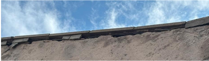
Figure 10 Showing gaps under the coping stone on the eastern gable end.
