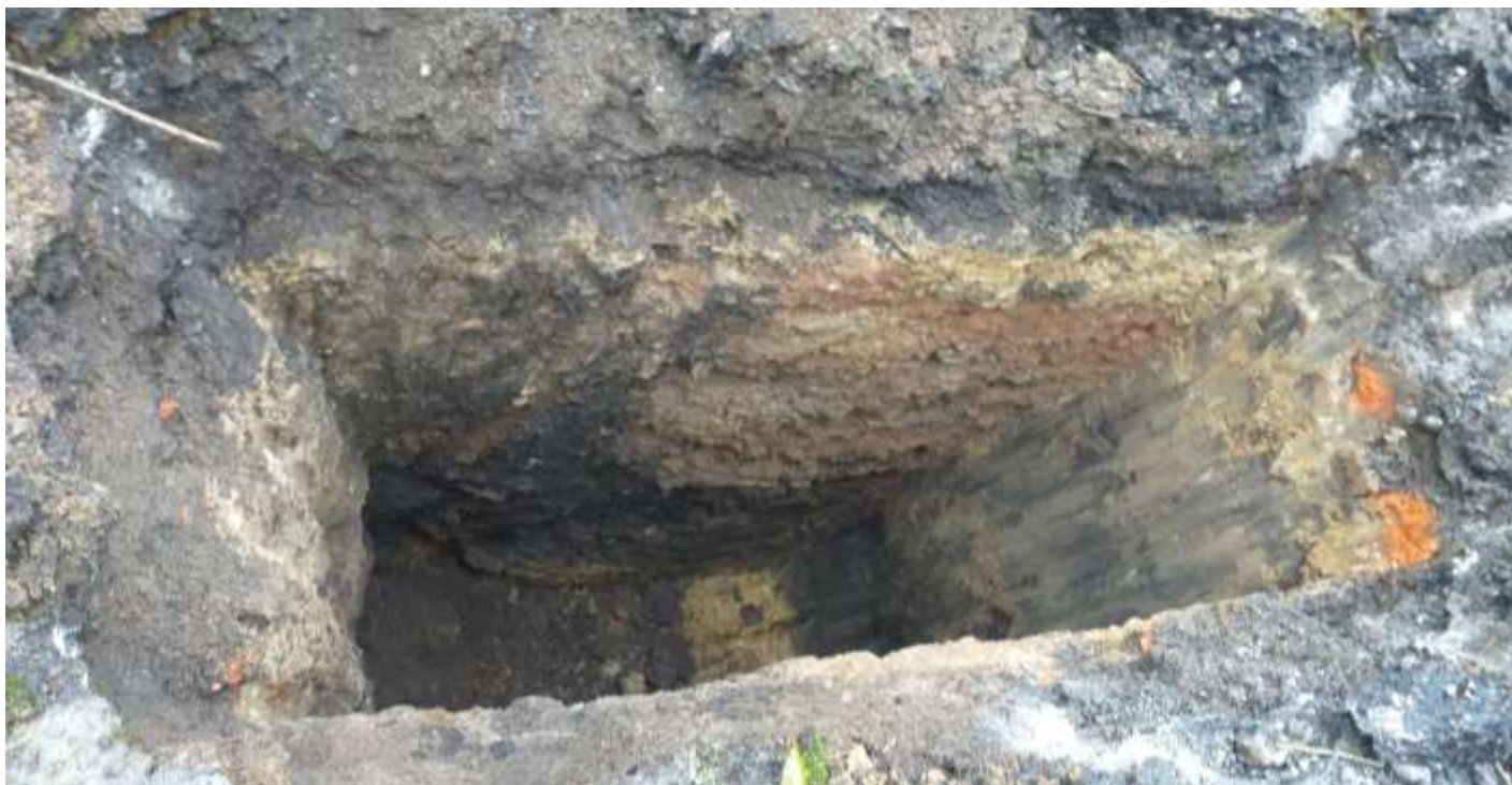
Photo 7: TP6 complete at 3.00mbgl.
