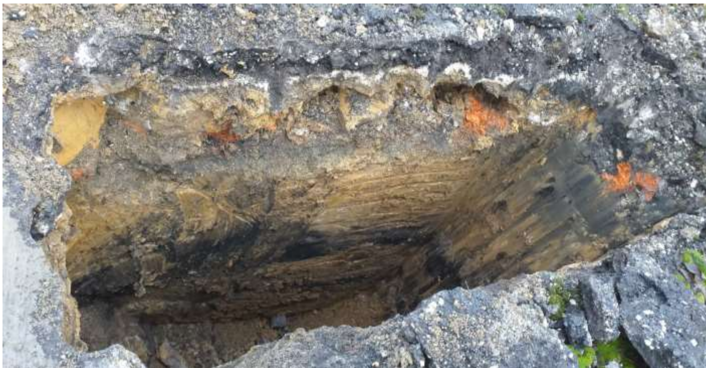
Photo 5: TP4 complete at 2.50mbgl.
