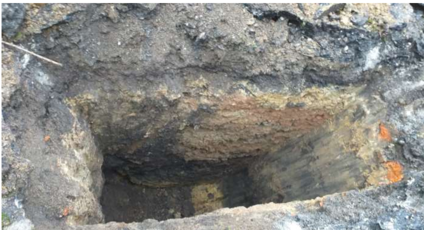
Photo 6: TP5 complete at 3.00mbgl.
