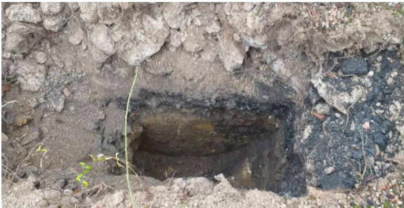
Photo 1: TP1 complete at 2.00mbgl.
