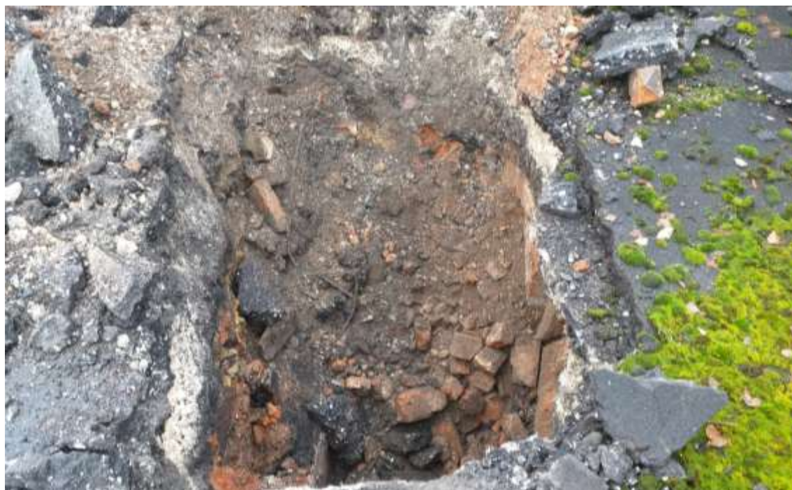
Photo 4: TP3 complete at 1.50mbgl.
