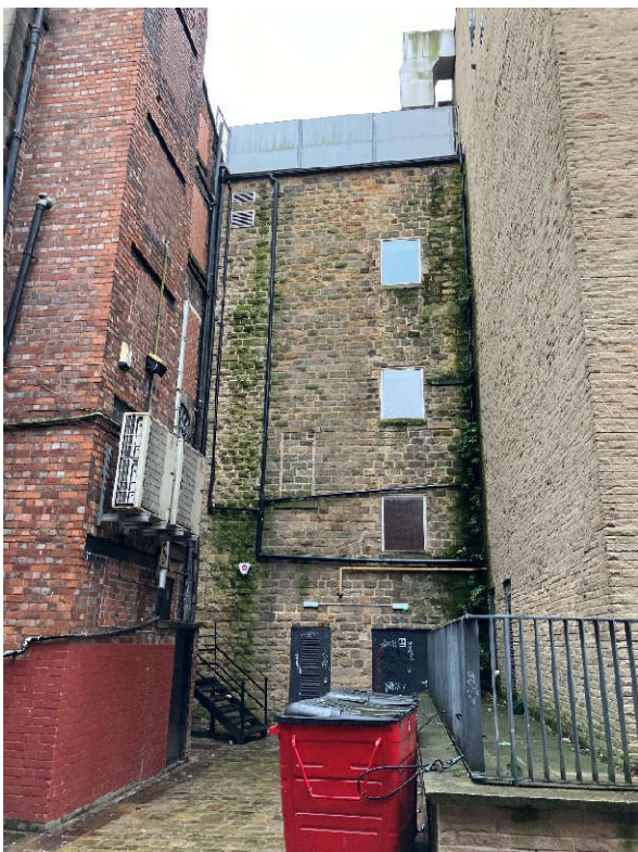
Fig 04. Part of original north elevation showing various alterations of original openings and addition of inappropriate services, pipework and clutter.
