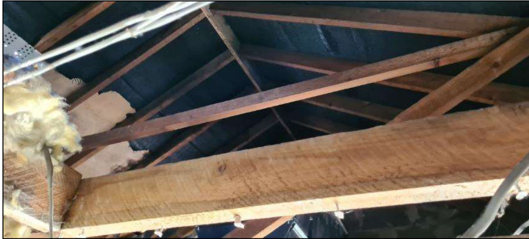
Plate 5. The loft space at the southern end of the building (looking up from the first floor)
