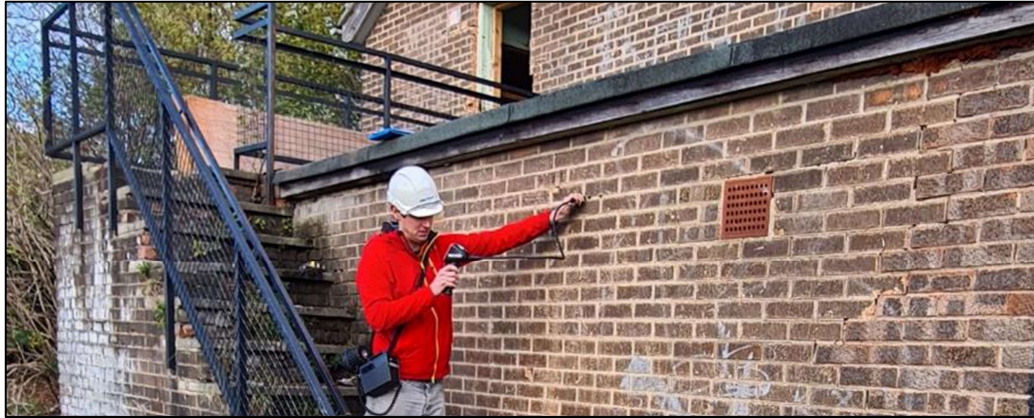
Plate 3. Inspection of a potential roost feature on the southern end of the building using an endoscope
