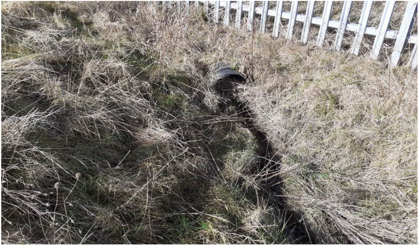
Plate 6: Small drainage pipe, to be blocked, raising the water table marginally, in order to make Receptor Area 3 more suitable for marsh orchids.
