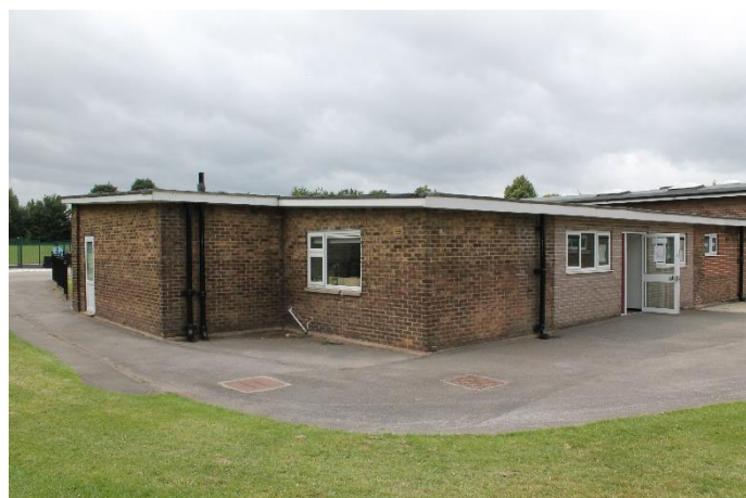
Adjacent classroom and corridor to proposed building footprint
