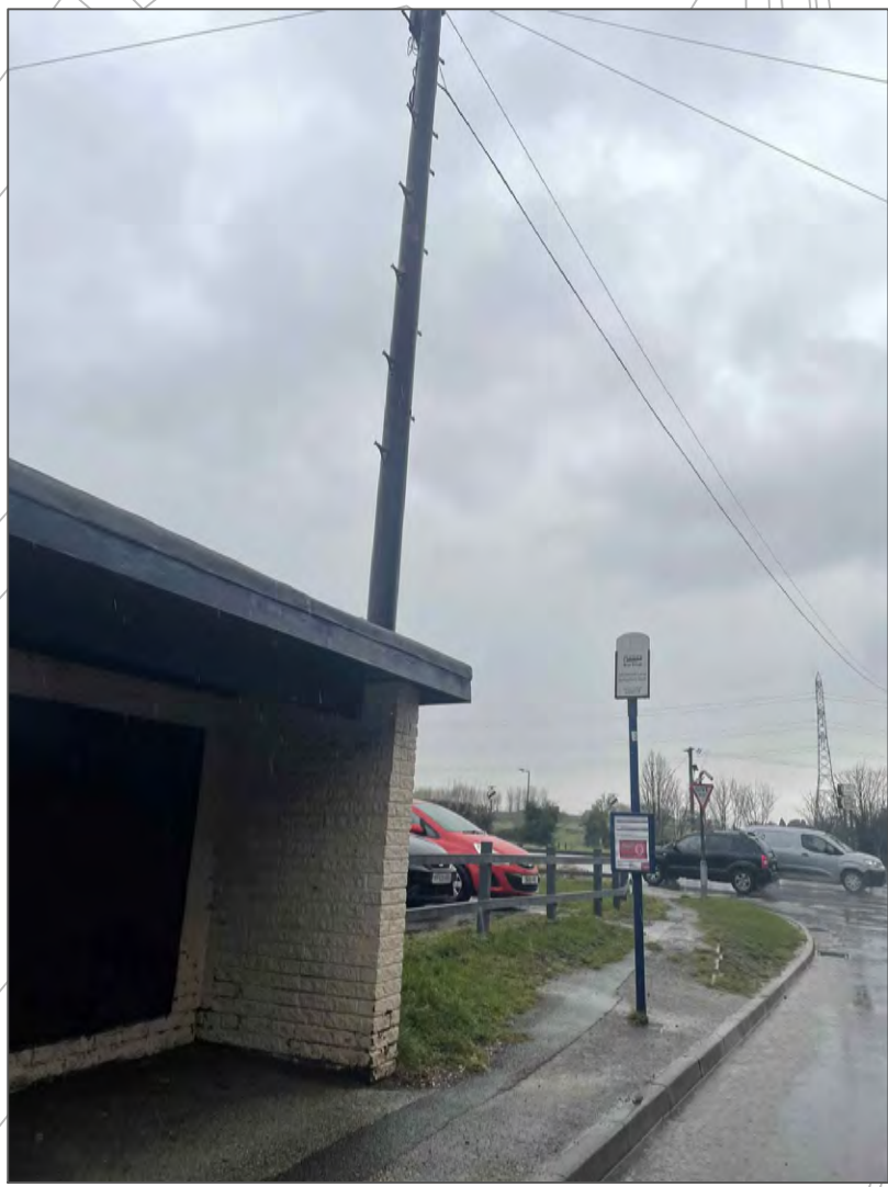
Bus shelter located along Middlecliffe Lane, accessible via footways – Photo taken facing North East
