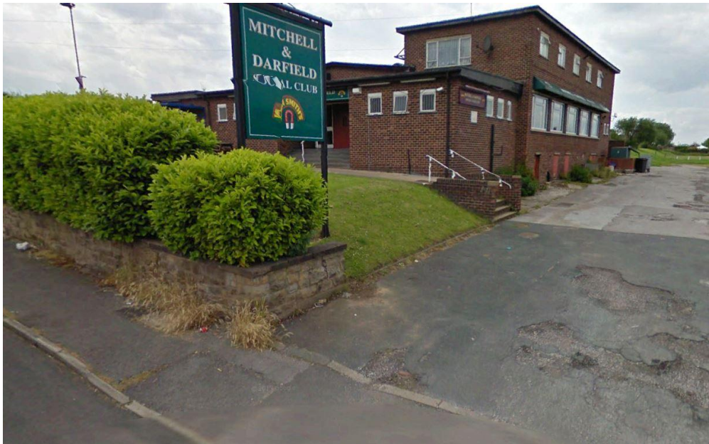
SITE AND EXISTING BUILDING FROM ROAD
