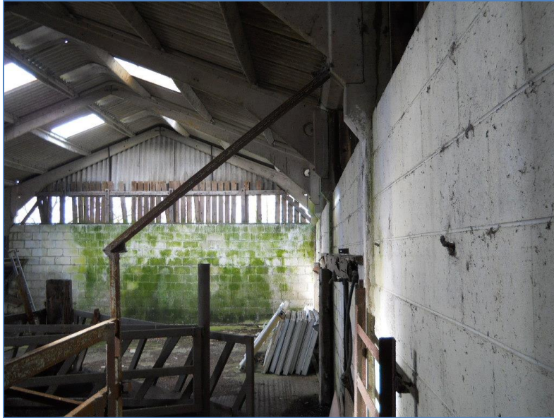
Figure 3: Far northwestern elevation of B3 interior - open access from tree line behind barn to barn interior for foraging bats.
