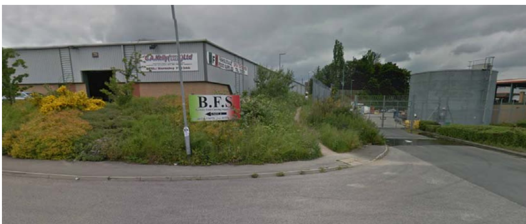
Pedestrian track from Fields Lane with B&Q service yard access and sprinkler tanks to the right
