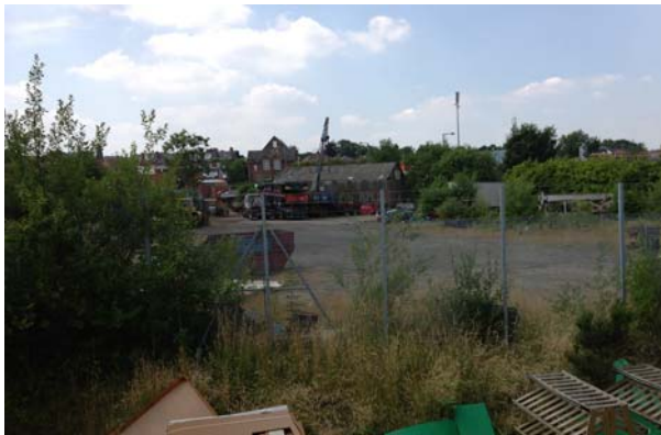
Industrial unit to west of the B&Q Garden Centre
