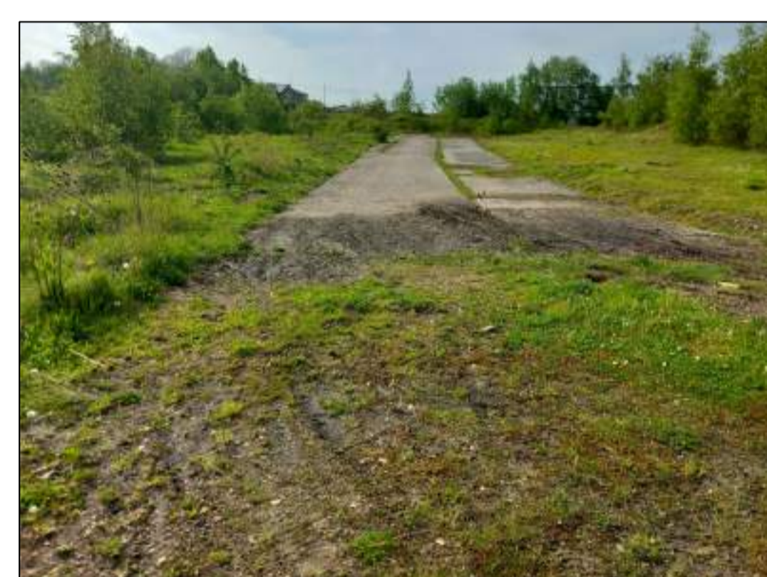
8. View south showing concrete slabs.
