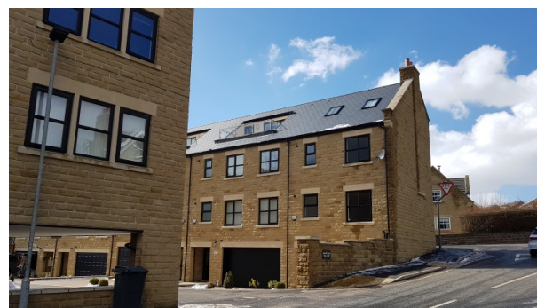
Inset roof terraces on the recent development corner of Green Road / Mortimer Road
