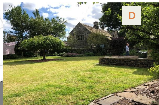
Existing view south-east to Willow House over site
