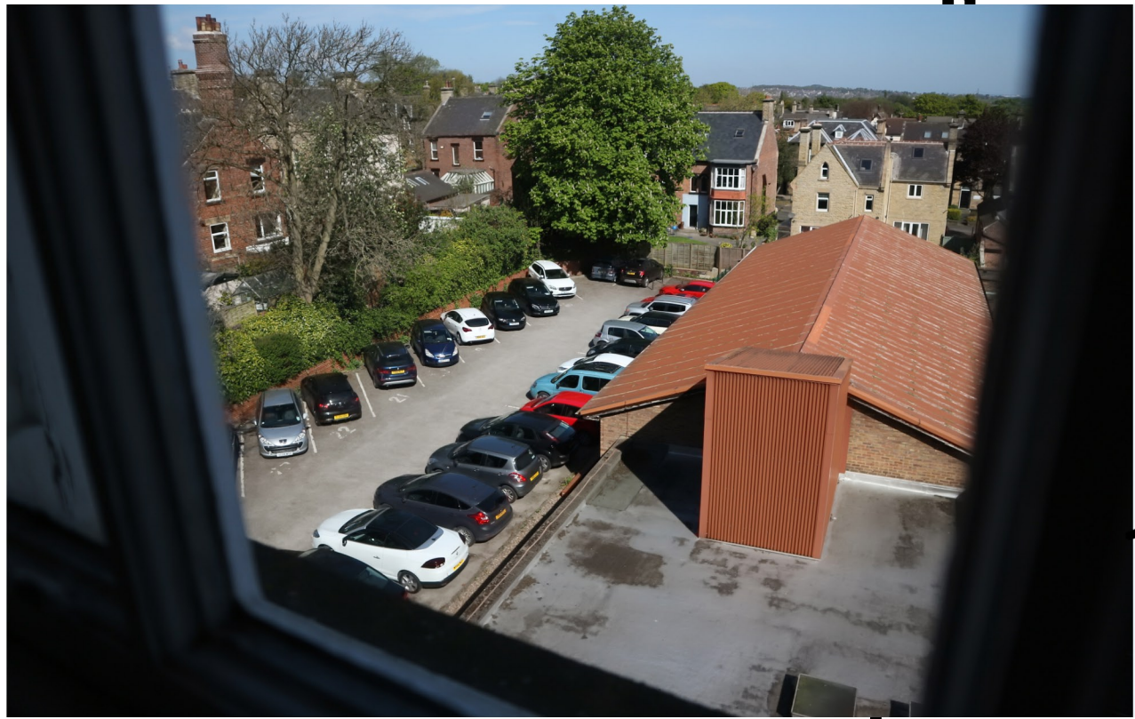
Existing retaining wall and car parking hard surface extents retained to north western boundary.
