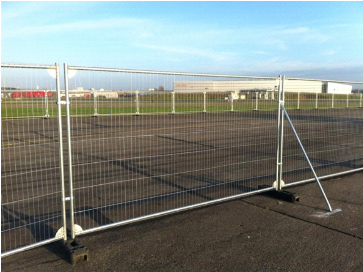
Heras tree protection fencing
