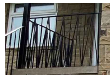
Existing External Balustrade
