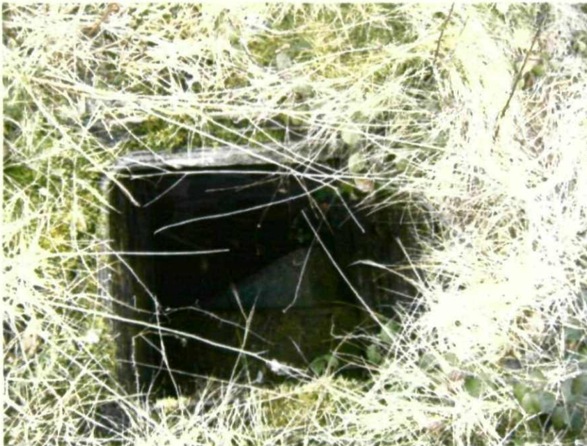
Photograph 18 – Showing old manhole.
