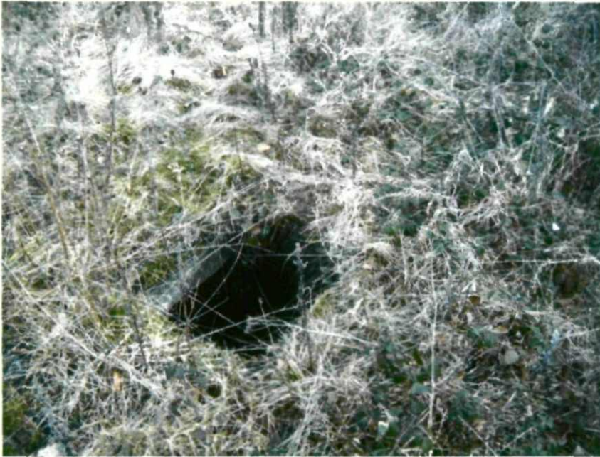
Photograph 17 – Showing old manhole.
