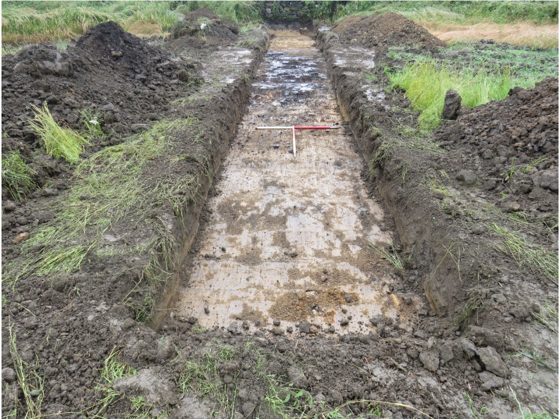
Plate 8. The southern half of Trench 9, viewed facing north-west towards the boundary wall. Scale 2 x 1m.
