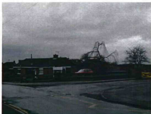
Site access & caretakers house
