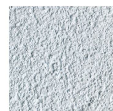
Smooth render finish to rear elevation panels
