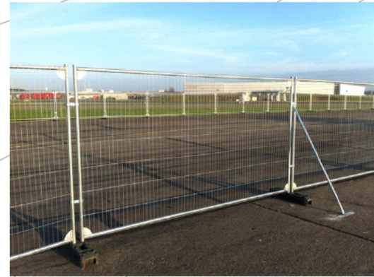
Heras tree protection fencing
