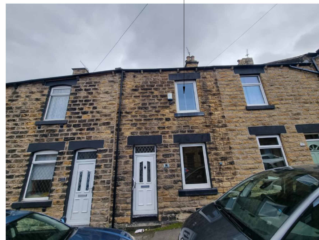
Replacement modern windows, stone head and cills
