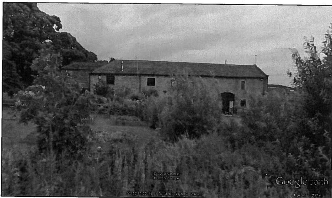
Western Elevation of Wellhouse Grange as viewed from Well House Lane
