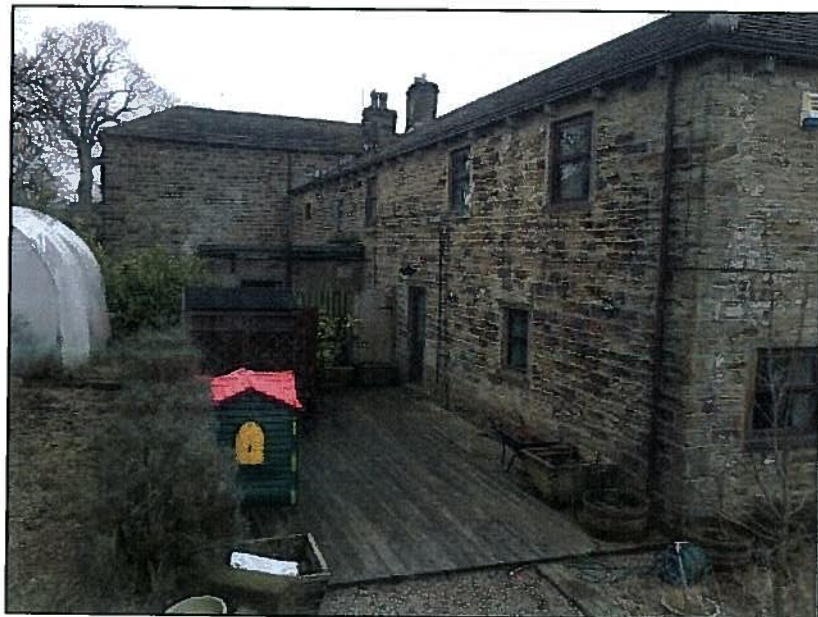
Photograph showing North Elevation and proposed location of extension – note the existing single-storey extension at adjoining property
